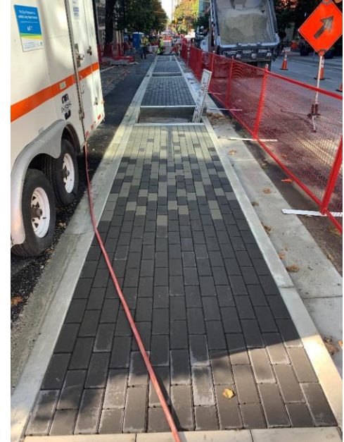
Block B - Permeable pavers with modified median width – no paver cutting
