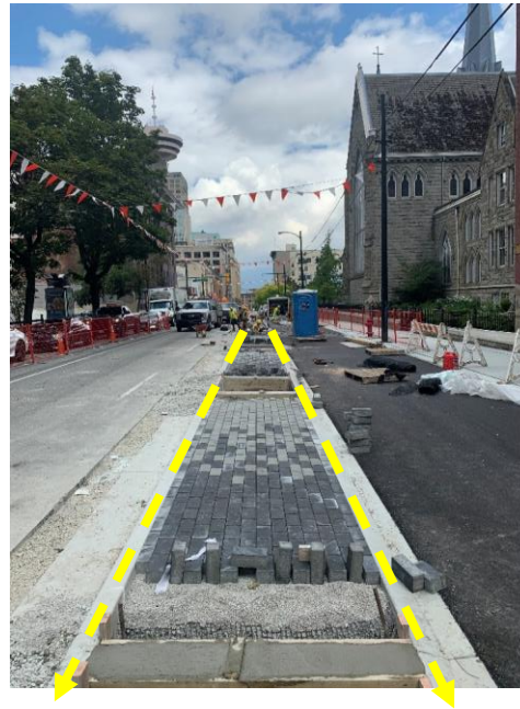
Block A- Permeable pavers with non-modified median width
