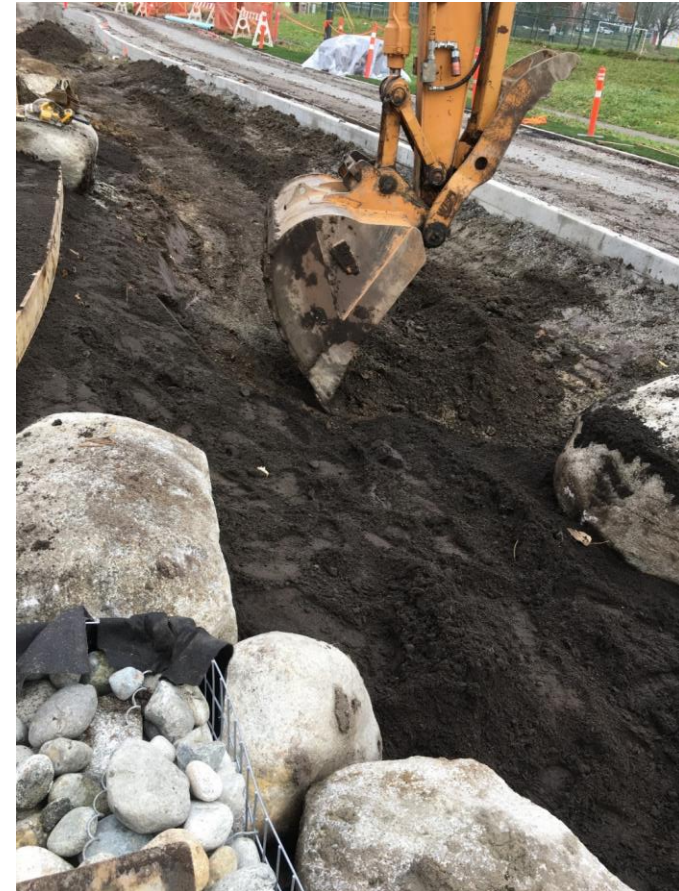
New growing medium being mixed with subsoil
