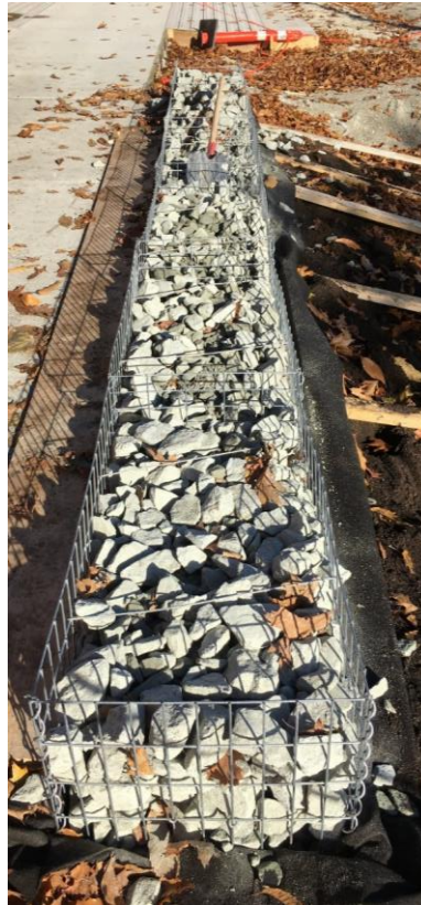
Gabion basket with 75mm clear crush
