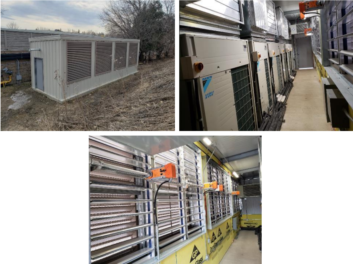
Figure 2-1. (Top left) Enclosure that houses outdoor units. (Top right) Inside view of enclosure showing heat pumps. (Bottom) Inside view showing dampers and gas unit heater.
