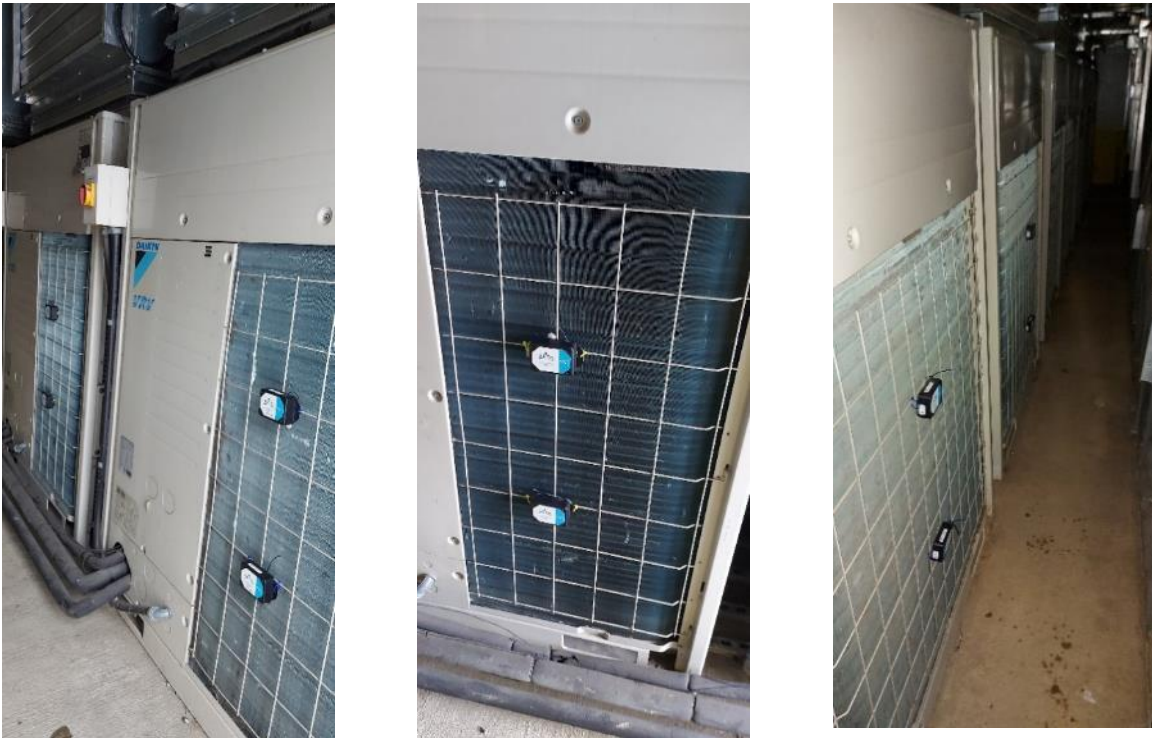
Figure 22-1. Temperature sensors were placed on the front, side, and rear grills, as well as the exhaust, of the two heat pumps forming the outdoor unit for the monitored subsystem.
