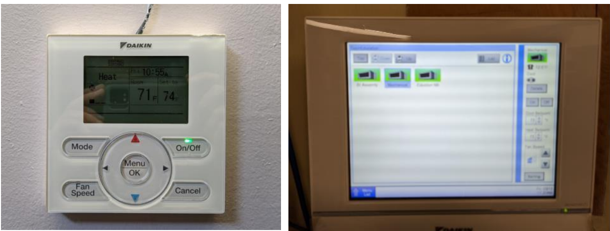
Figure 2-2. (Left) Navigation Remote Controllers provide local controller for the indoor fan coils. (Right) The intelligent Touch Manager provides central control and a user interface for the system, as well as being the BACNet interface for the Johnson Controls building automation system.
