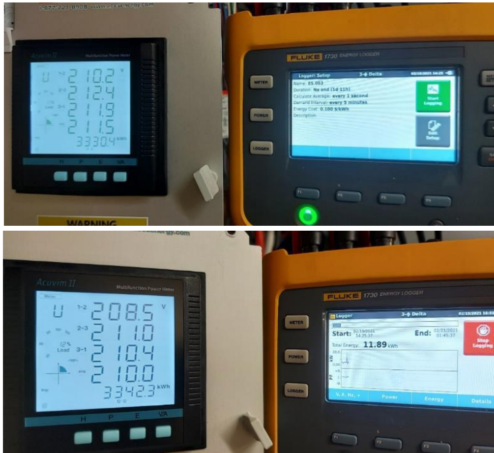
Figure 19-1. A Fluke 1730 Energy Logger was used to verify the electricity consumption measurements of the Acuvim II meter.
