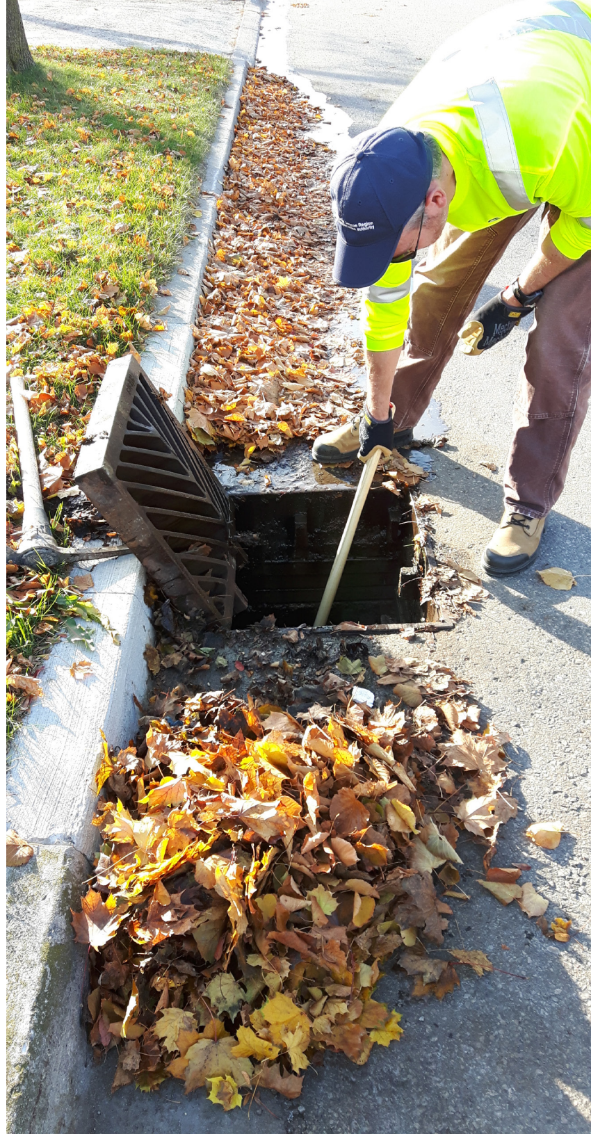
Figure 6- Removal of a CB Shield from a catch basin
