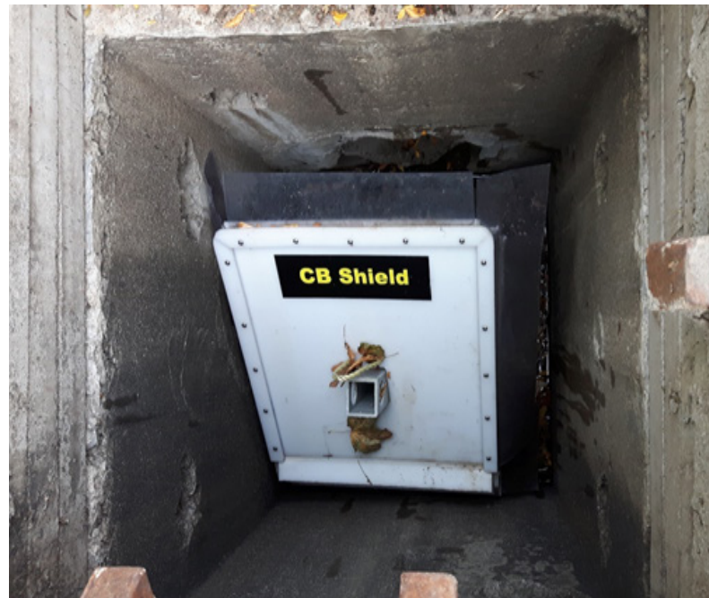
Figure 1 – Example of a CB Shield installed in a typical catch basin
