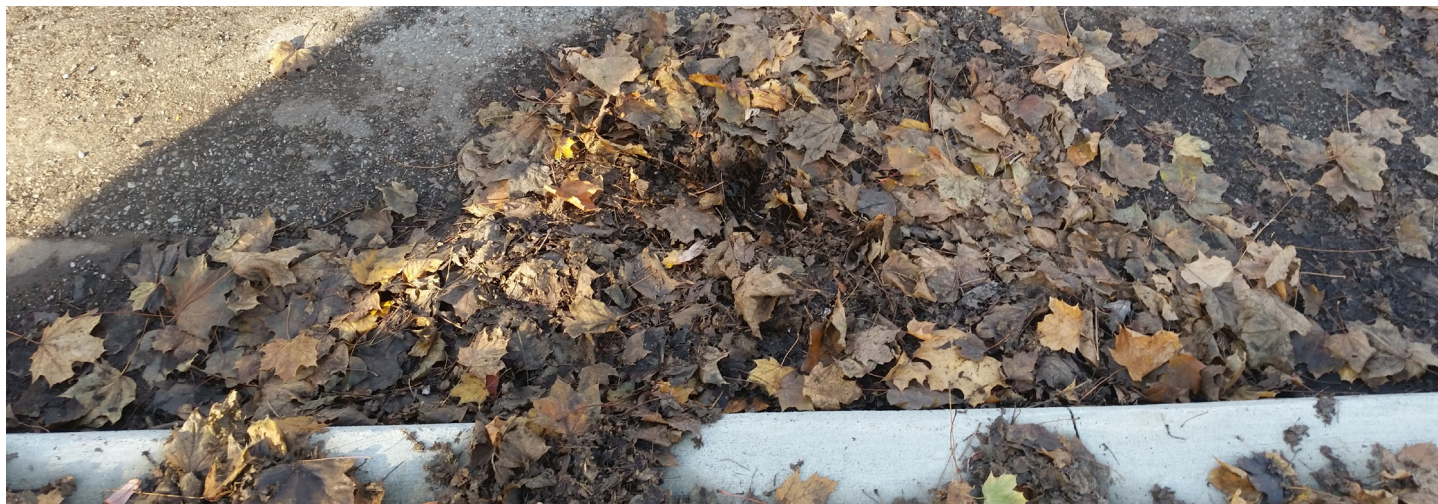
Figure 7- The top grate of a catch basin completely blocked by accumulated leaves, grass clippings and sand
