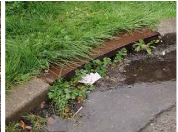
Inlet clogging, requires re-design of pre-treatment
