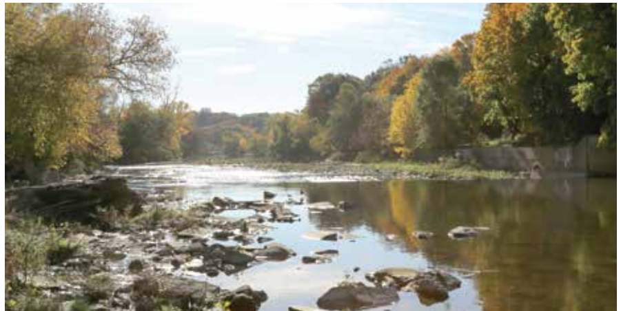
Stormwater retention ponds can be significant contributors to thermal enrichment of streams.
