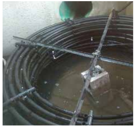
L to R: Figure 1. Schematic diagram of the pilot geothermal stormwater cooling system. The coil of high-density polyethylene pipe used as the stormwater heat exchanger (SHX) in the geothermal cooling pilot.
