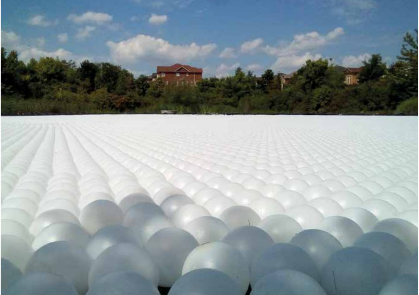
Hollow, high-density polyethylene balls cover the surface of the Esker stormwater management pond in Brampton, Ontario.
