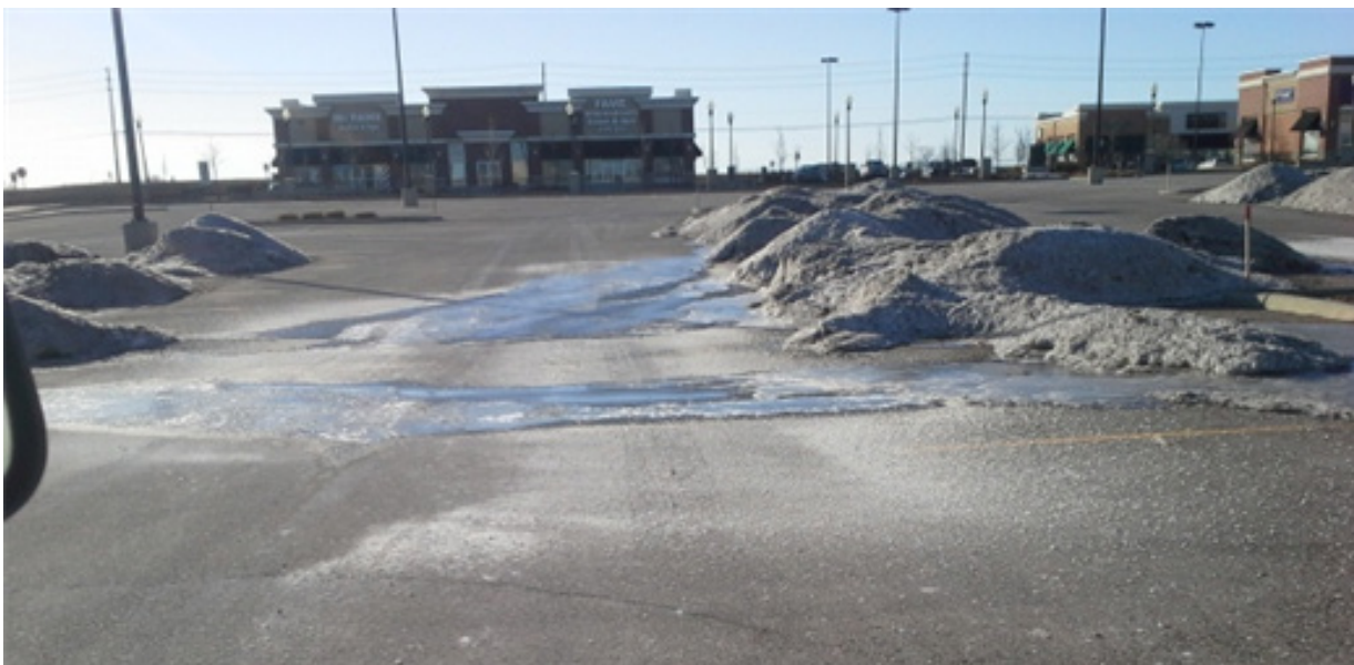
Figure 6 An example of a trouble spot due to freeze/thaw from improperly placed snow piles
