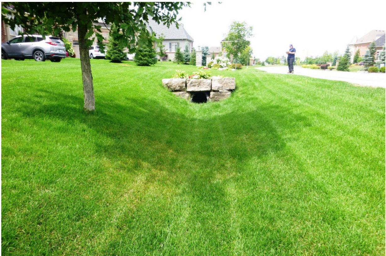
Figure 23: Example of a grass swale that appears to be regularly maintained by resident.
