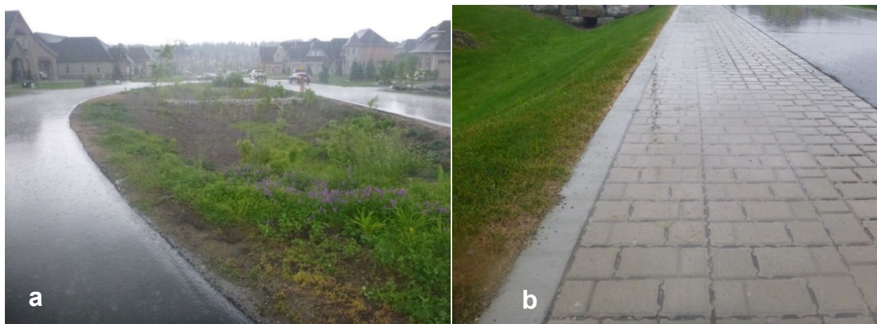
Figure 4: a) Bioretention cell during a rainstorm; b) Permeable pavement and grass swale during a rainstorm.
