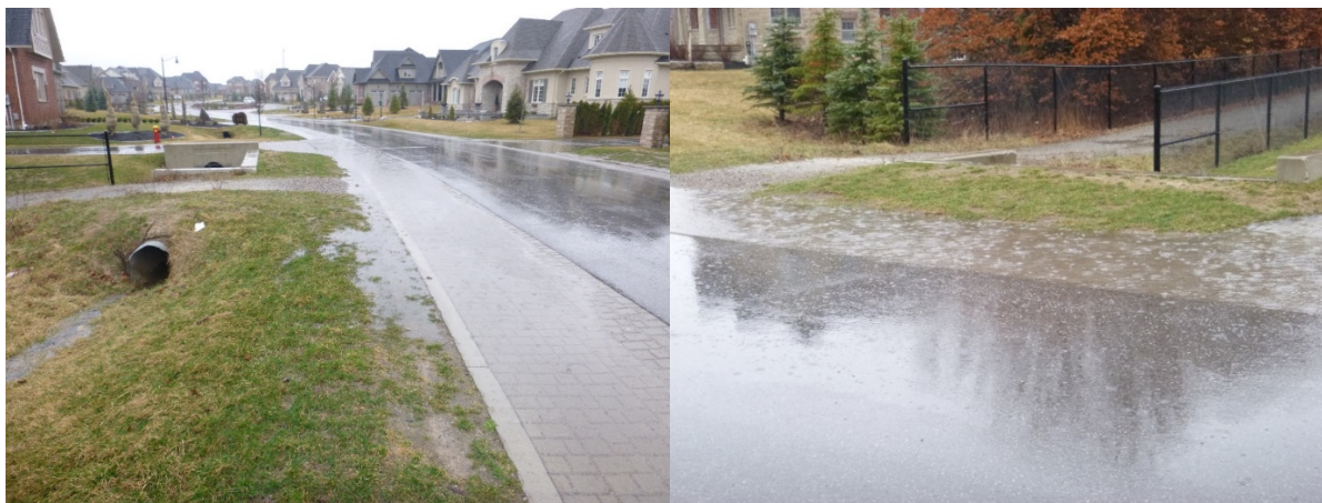
Figure 24: Permeable pavement across the road from Inlet 1, shown during a precipitation event.
