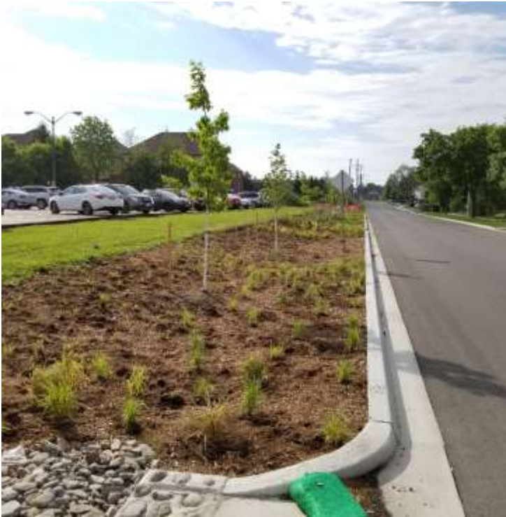
Tested a new approach – CU Soil Base Layer and Topsoil Upper Layer
