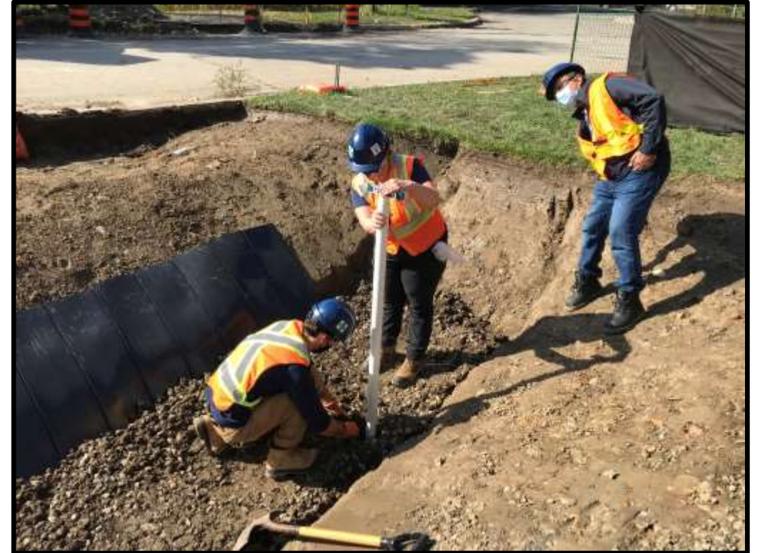
Monitoring Well Installation
