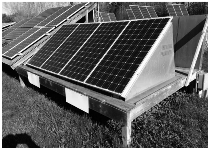
Figure 3. Four modules were mounted with ballast on a flat deck.
