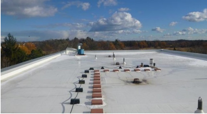
Figure 5. CVC's concrete slab roof
