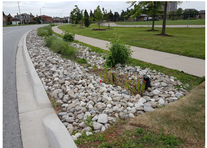
Figure 6: Curb inlet at the bioretention
