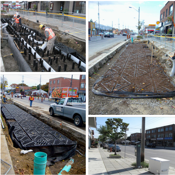
Figure 4. Soil cell construction and final planting (source: P. Cheung)
