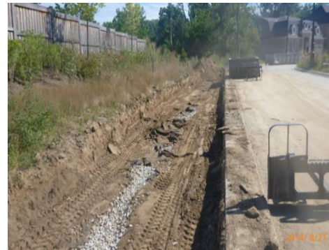
Figure 3: Rehabilitation of bioswale. Source: CVC
