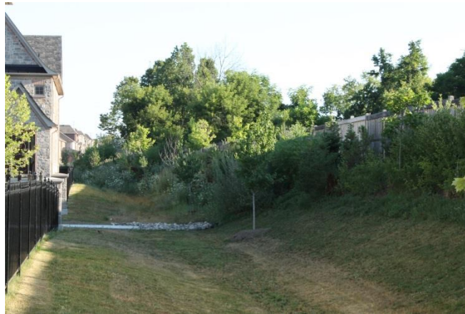
Figure 3-9: Bioswale
