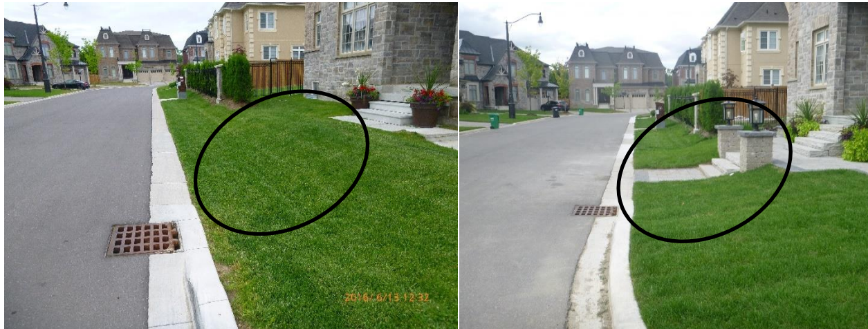
Figure 5: Resident walkway constructed through grass swale. Source: CVC
