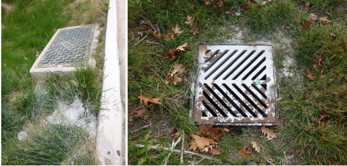
Figure 4-35 and Figure 4-36: Truck washout near rolled curb and overflow catch basin June, 2016 and signs of possible truck washout near catch basin in December 2017.
