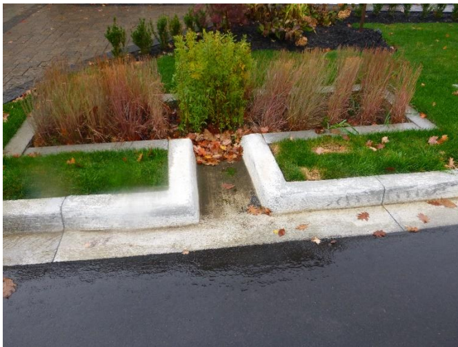
Figure 4-47: Rain Garden 90-degree inlet, bypass observed
