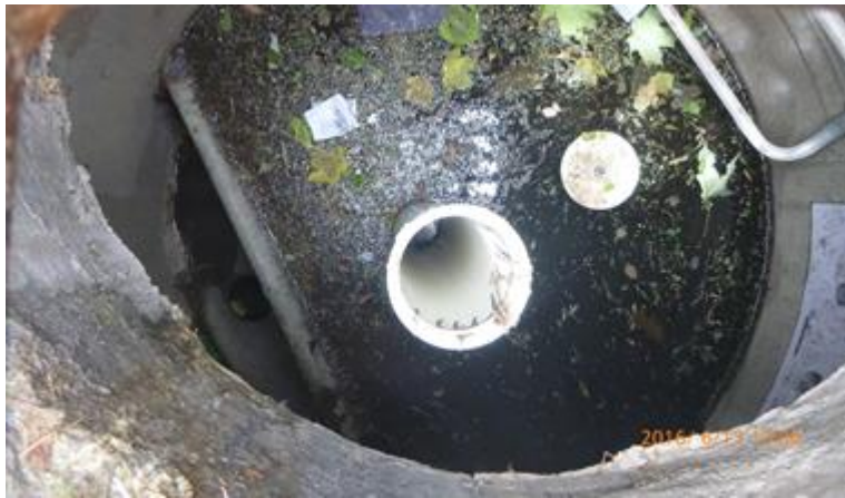
Figure 4-42: OGS clogged with sediment and grass clippings in June 2016
