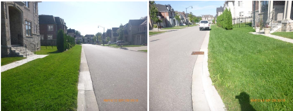
Figure 4-13: Rolled Curb Inlets to enhanced swale and catch-basin location
