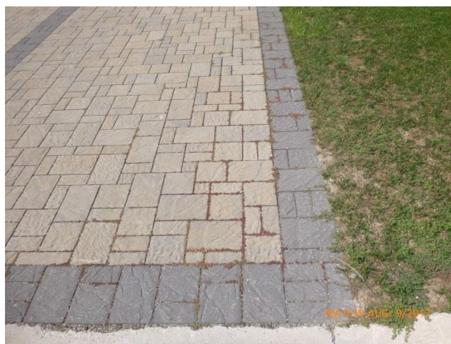
Figure 4-30: Permeable Pavement Partially Blocked with Weeds in August 2017
