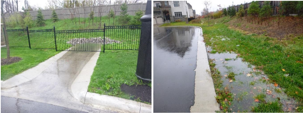
Figure 4-12: Curb-cut and Rolled Curb Inlets to Bioswale
