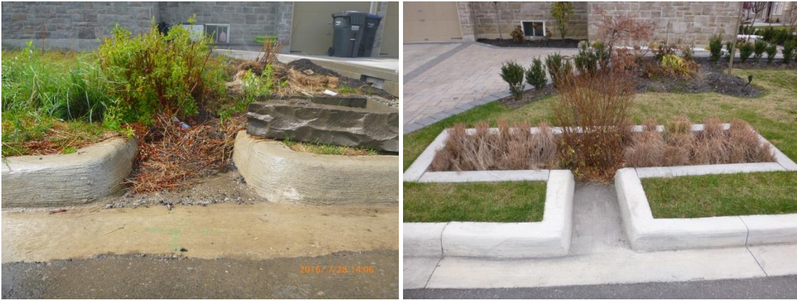
Figure 4-38 and Figure 4-39: Rain Garden Inlet (with debris and sediment accumulation and without impediments) in July 2016 and November 2016.
