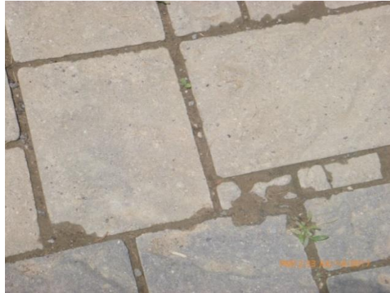
Figure 4-28: Close-up of Permeable Pavement Blockage, July 2017
