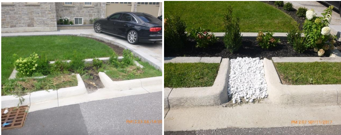
Figure 4-40 and Figure 4-41: Rain Garden Inlet (clogged with sediment prior to gravel installation and inlet modified by home owner) in July 2017 and September 2017.
