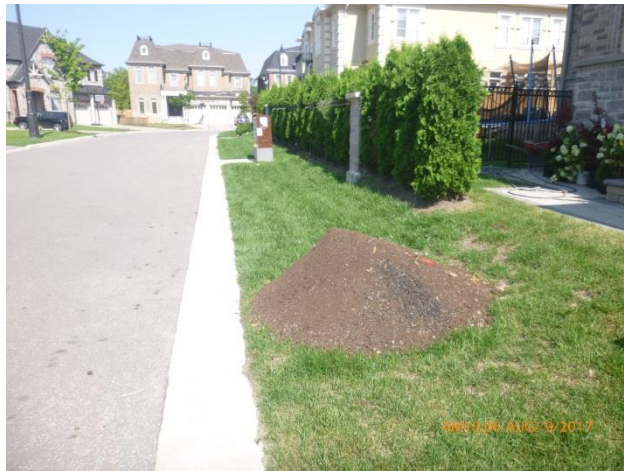
Figure 4-37: Excess soil material left in grass swale in August 2017
