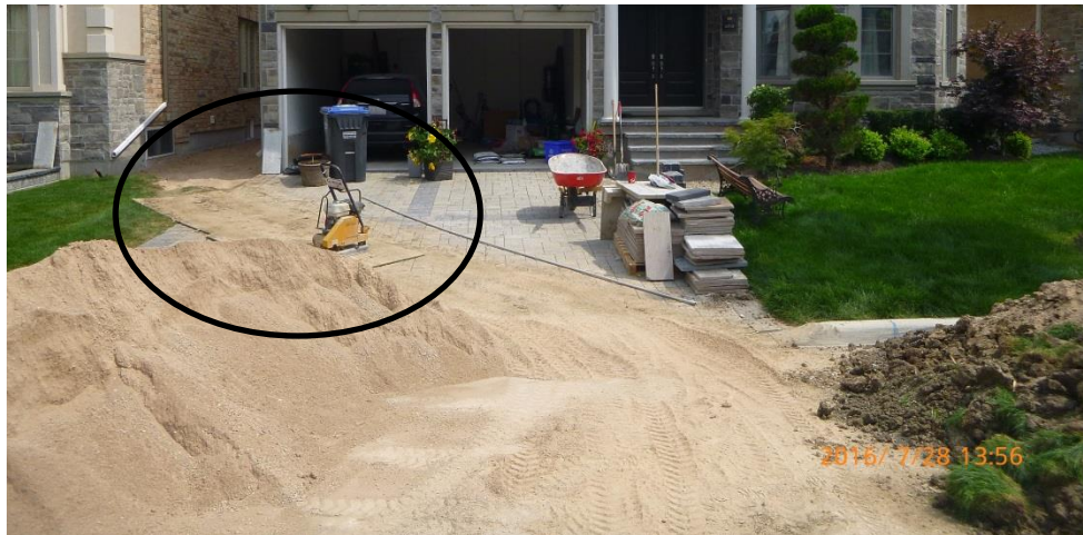
Figure 4-29: Permeable Pavement Blocked with Construction Materials in July 2016
