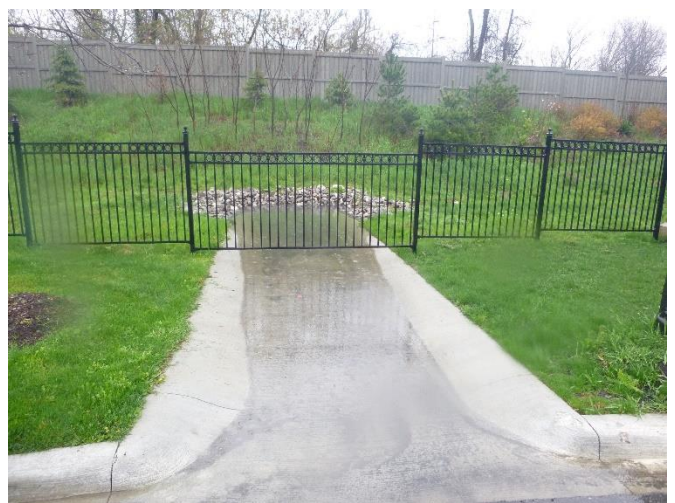
Figure 4-48: Example of wide curb cuts from bioswale
