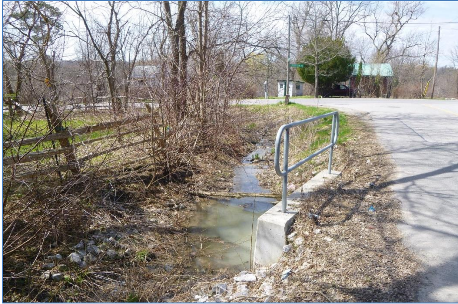
Figure 3-12: Outfall headwall and downstream receiver
