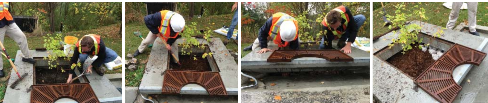
Figure 7. Maintenance of the Filterra® unit
