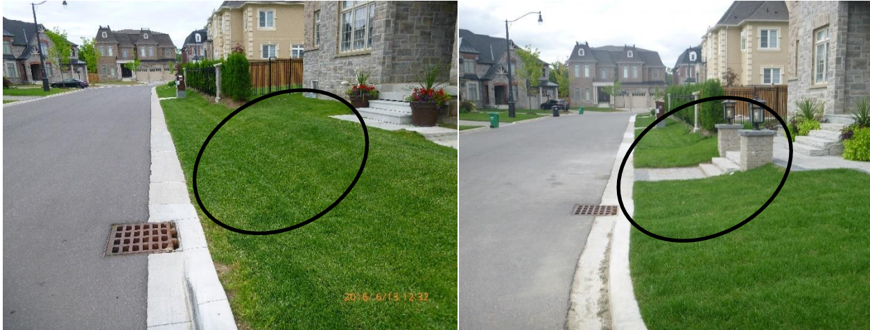
Figure 5: Resident walkway constructed through grass swale. Source: CVC (2016)
