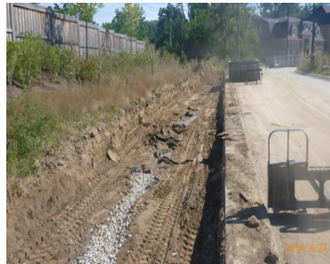
Figure 3: Rehabilitation of bioswale. Source: CVC (2015)
