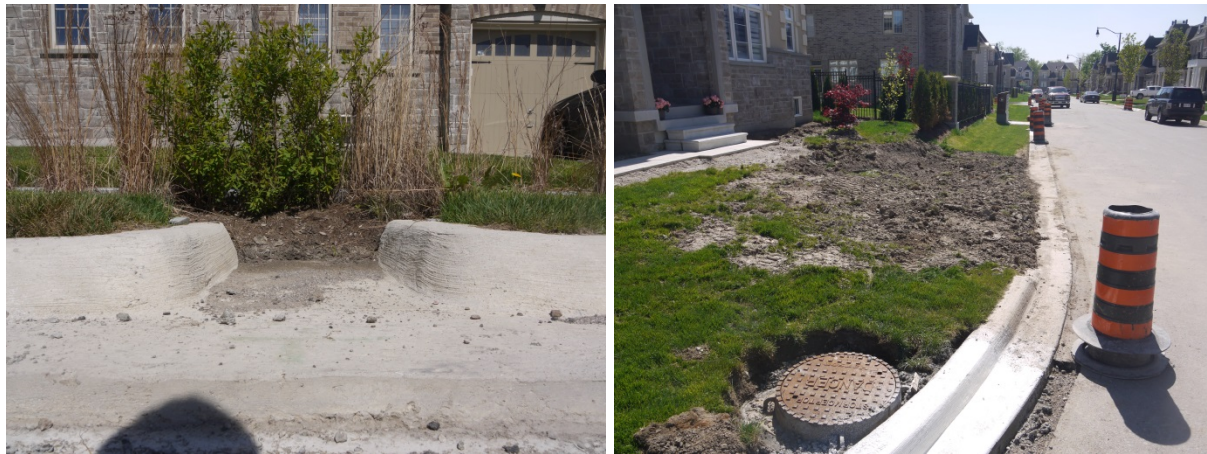
Figure 5 Rain garden with finished curb with respect to media grade (left) and impacted rain garden due to adjacent construction (right)
