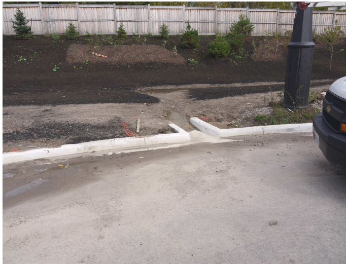
Cul-de-sac on Fairmont Close – there is fine construction debris accumulating in front of the inlets to the bioswale (this could clog and/or reduce the performance of the system)
