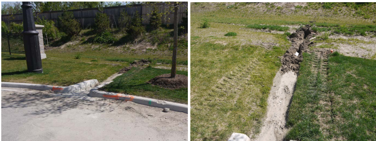
Figure 4: Preparation of inlet for construction
