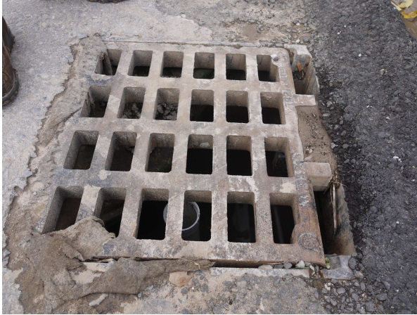
Catch basins are missing, or have damaged geotextile fabric
