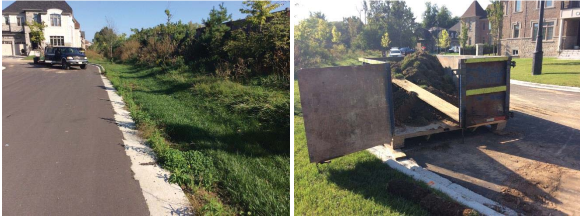
Figure 1: Bioswale with sod bin nearby
