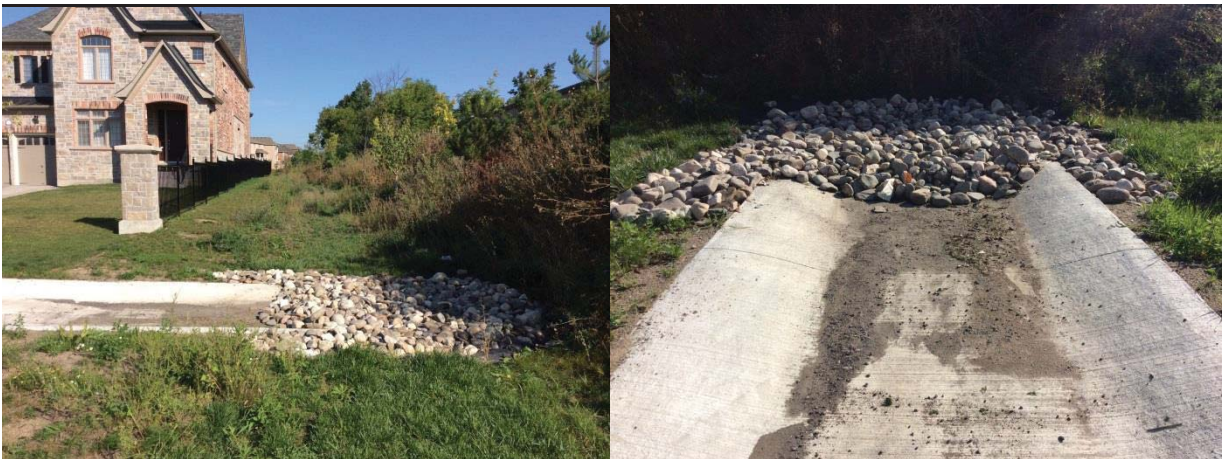
Figure 2 Sediment Buildup within Inlet
