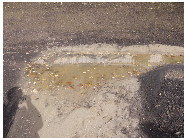
We observed some ponding at the inlet and in the puddle in the background of this photograph. Ponding water can mean that the bioretention soil media is becoming clogged with fine debris and is not draining properly.
