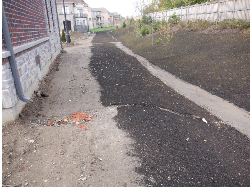
Washout of mulch is occurring because the flow from the downspouts is not being spread out by a splash pad and by sod.
