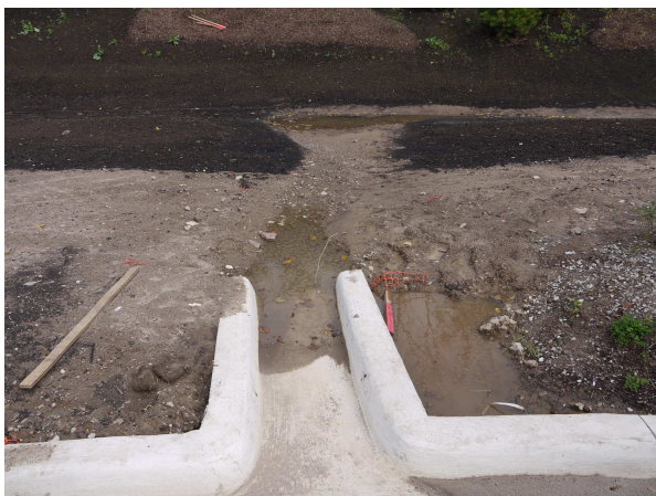
We observed some ponding at the inlet and in the puddle in the background of this photograph. Ponding water can mean that the bioretention soil media is becoming clogged with fine debris and is not draining properly.
