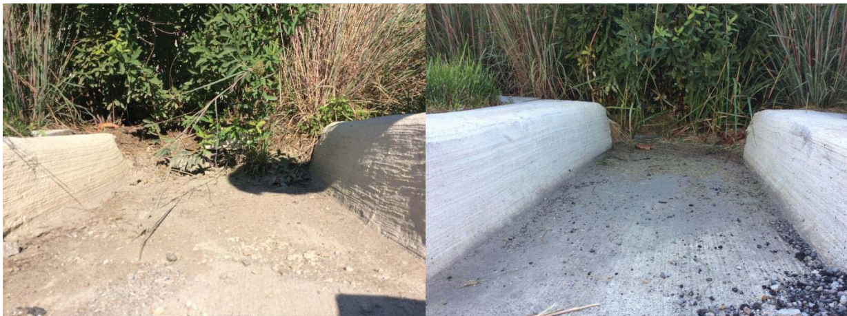
Figure 4: Rain Garden inlets blocked with high soil, plantings, mulch
