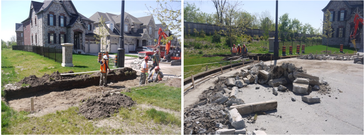
Figure 3: Replacement of existing inlets
