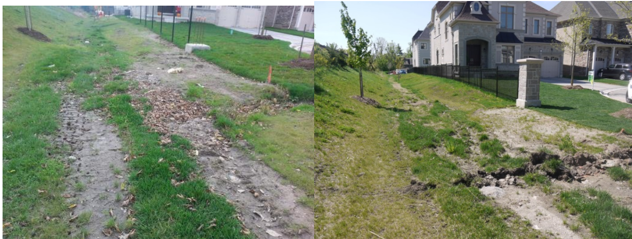
Figure 2 Sediment Buildup Downstream of Inlets. Oct 9, 2014 Left. May 15, 2015 Right.
