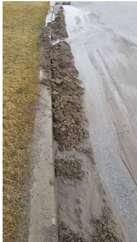
Sand accumulates on the side of the road
