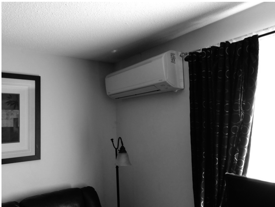
Figure 3. Wall-mounted indoor fan coils were used but ceiling- and floor-mounted options are also available
