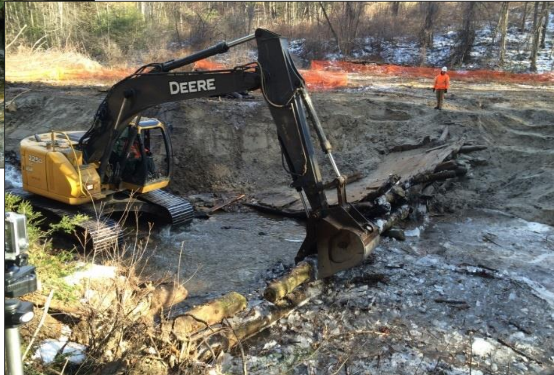
Timber Dam Removal January, 2016
