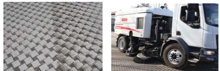
Figure 5. Pavement before maintenance and vacuum sweeper in action.
