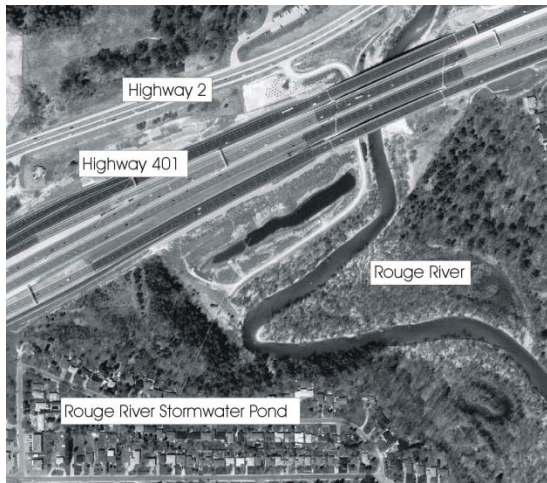
Figure A 1: Rouge stormwater management pond
