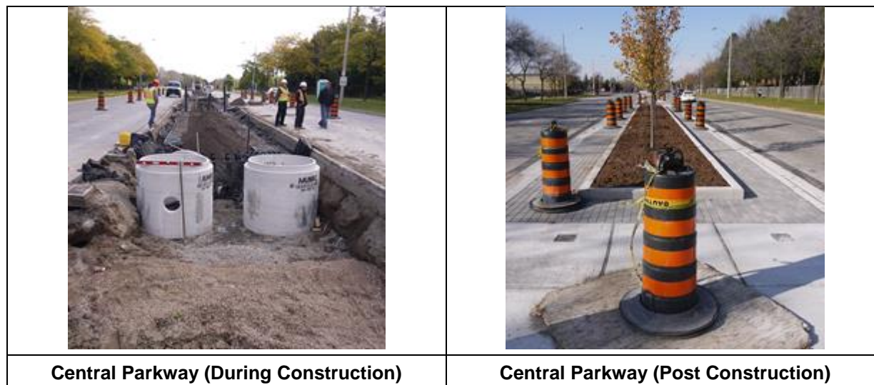
Figure A 4 Road right-of-way (ROW) retrofit example using a pre-cast silva cell system
