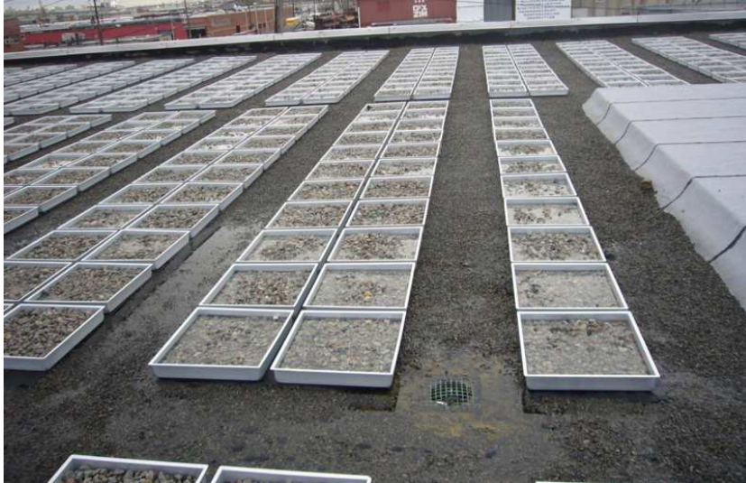
Figure 4: An example of a modular tray blue roof. Source: Massachusetts Department of Environmental Protection
