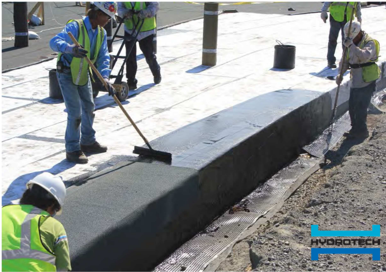
Figure 20: Installation of liquid applied membrane (American Hydrotech Inc)
