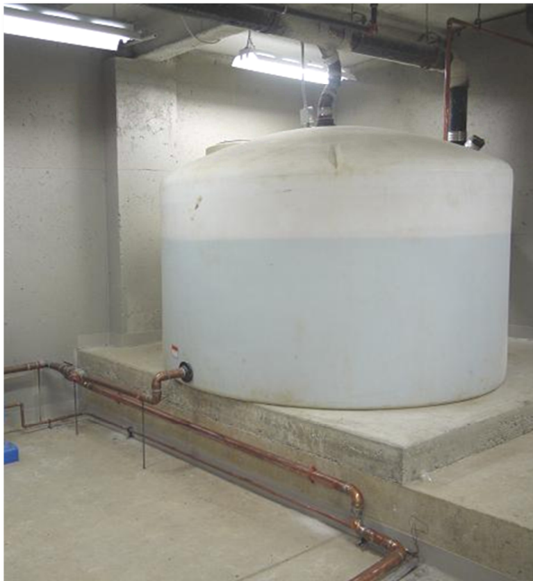
Figure 11: Rainwater harvesting system located in the basement of Building A
