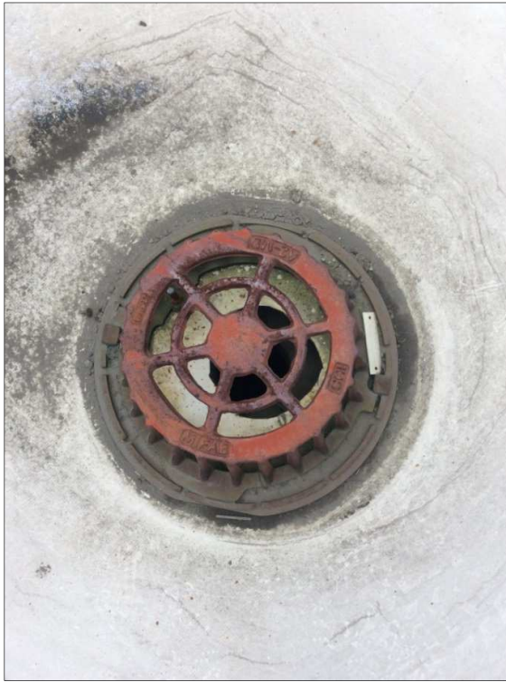
Figure 8: Building A - 100mm Roof Drain Inlet
