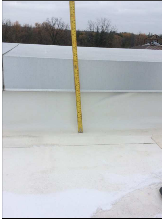
Figure 9: 450mm Perimeter roof lip without scupper
