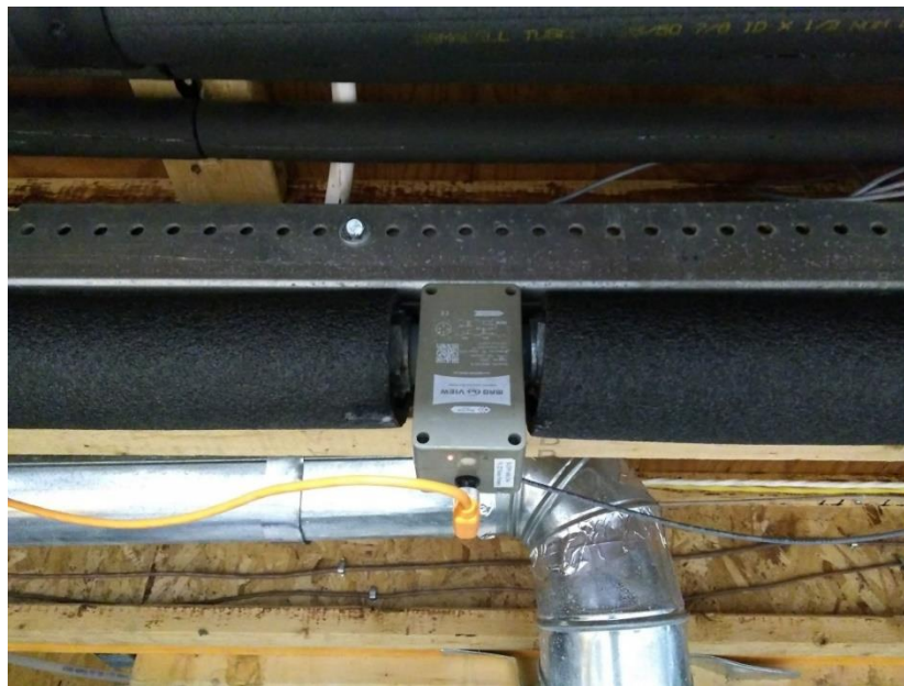
Figure 4-3. The primary loop magnetic flow meter was mounted in the basement of House B.
