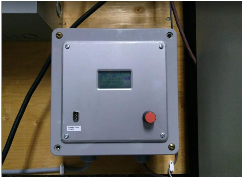
Figure 5-1. The DDC was used to input parameters for the GHP.
