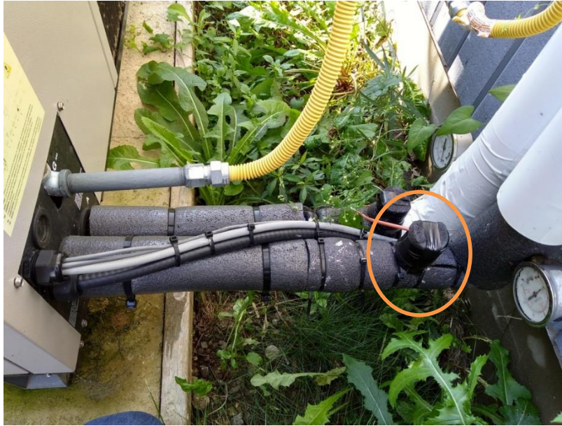
Figure 4-2. Supply and return temperature sensors were mounted as close to the unit as possible. They were mounted in thermal wells using a thermal grease and insulation was used to cover the thermal well.
