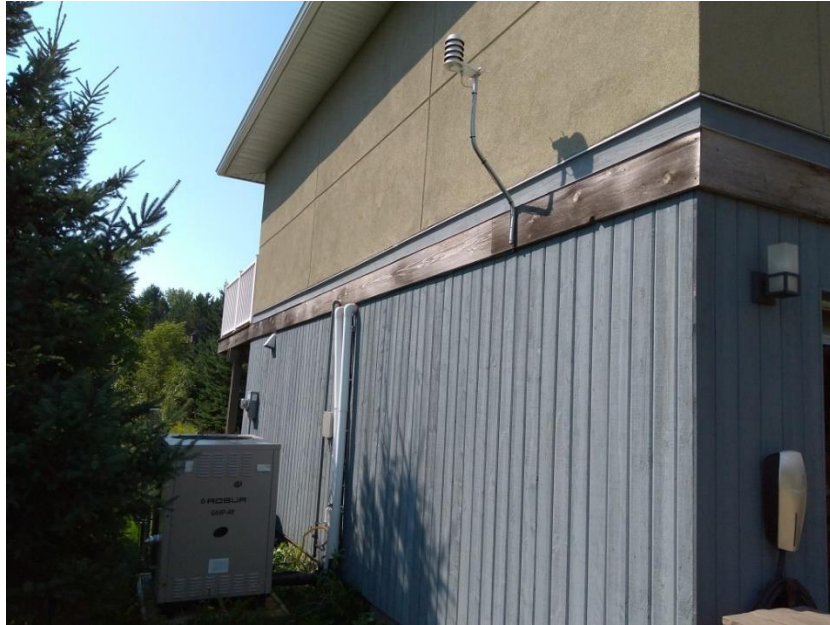
Figure 4-4. The outdoor ambient temperature and humidity sensor was installed with a radiation shield on the east side of the ASH roughly 12 ft (horizontally) from the GHP.
