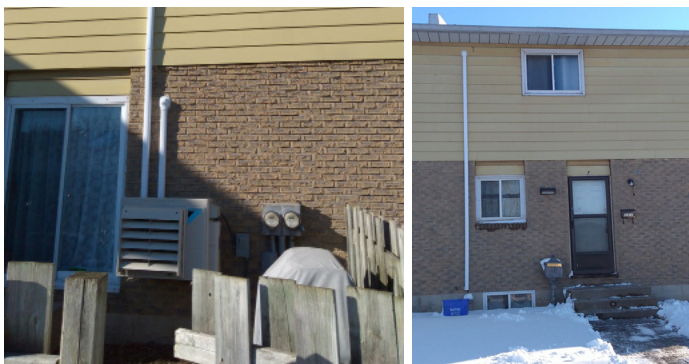
Figure 2. Outdoor coils were mounted in the back yard (left). Front bedroom fan coils were reached by routing refrigerant lines through the basement ceiling and then on the front exterior (right). This reduced the need for interior finish work.
