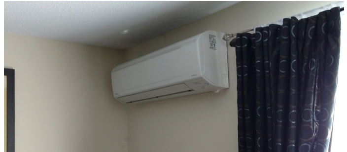
Figure 3. Wall-mounted indoor fan coils were used for an easy retrofit, although different indoor fan coil options, including floor-mount or recessed ceiling-mount, are possible.
