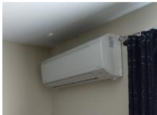
Figure B. Wall-mounted indoor fan coils were selected for this retrofit. Ceiling- and floor-mounted fan coils are also available.
