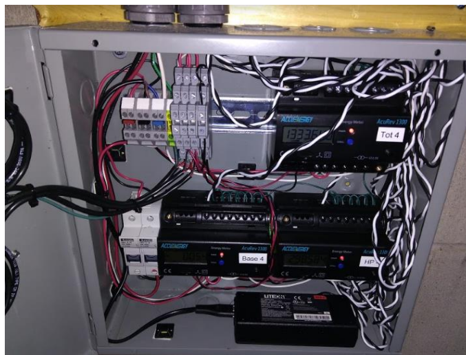
Figure 5-2. Close-up of a submetering box in a retrofitted rowhouse unit.
