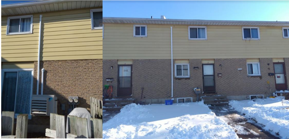
Figure 3-3. (Left) Outdoor coil and refrigerant line set for the Daikin heat pump mounted in the 2-bedroom rowhouse unit. (Right) Refrigerant line set was run through the basement and then on the exterior at the front of the house to reach the front bedroom.
