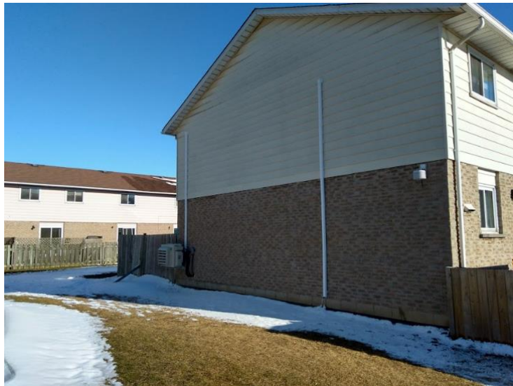
Figure 3-2. Outdoor coil and refrigerant line set for the Daikin heat pump mounted in a 3-bedroom rowhouse end unit.
