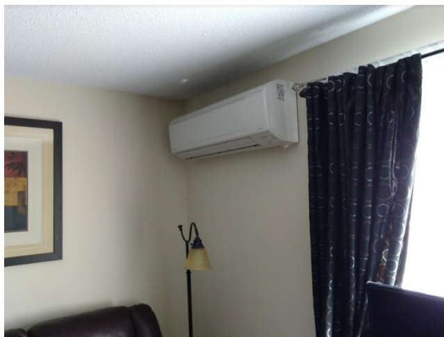
Figure 3-5. All indoor fan coils were wall-mounted with the return near the ceiling.
