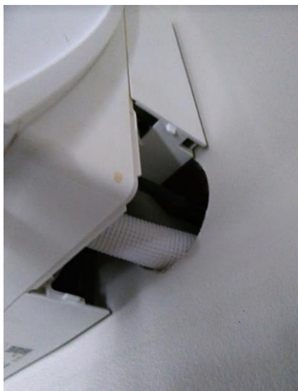
Figure 3-7. When the plastic cover was removed it was clear that the building penetrations had not been sealed by the contractor. This affected all of the baseline period and part of the retrofit period but is not believed to be a source of error since Figure 3-8 shows that the lack of sealing did not impact heat pump energy consumption.
