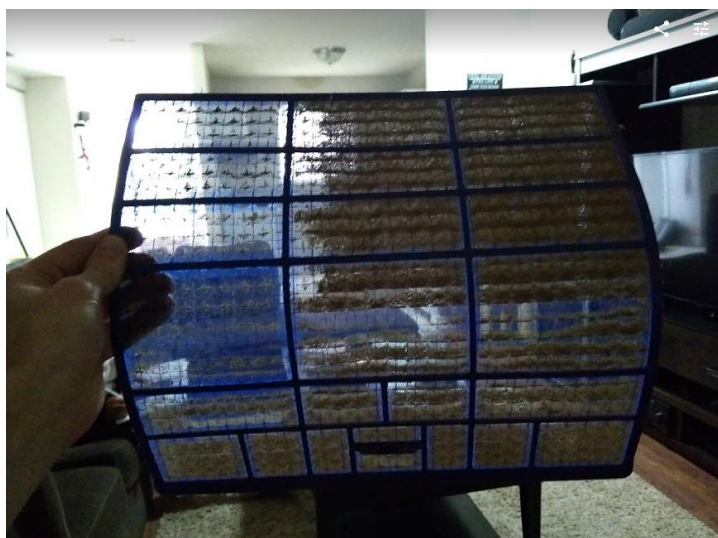
Figure 9-1. The Unit 2 filter was heavily soiled after 6 months of operation without a cleaning. The upper left part of the filter had been cleaned to illustrate what a clean filter ought to look like.
