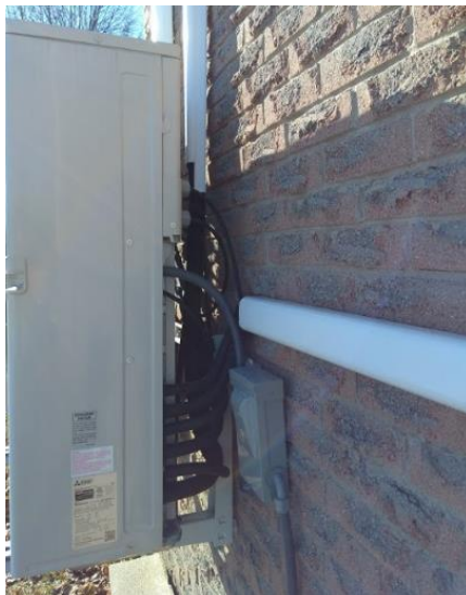
Figure 3-6. Refrigerant line sets were routed behind the outdoor coil for the sake of appearance but this would have also introduced parasitic heat loss from the lines.
