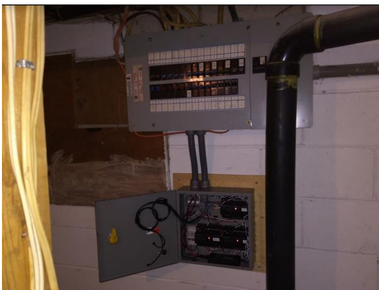
Figure 5-1. Electrical submetering boxes were installed adjacent to the main service panel.
