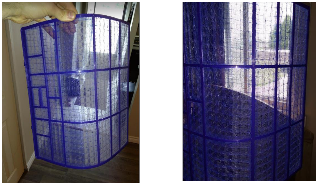
Figure 9-3. The Unit 4 filters showed a minimal amount of dust after 6 months of operation and this is not believed to have impacted the energy savings calculations for this unit.
