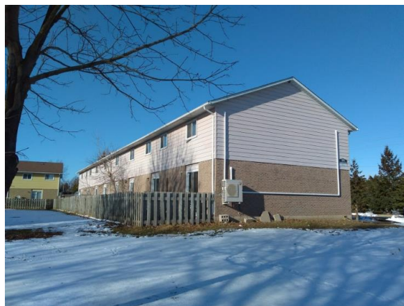
Figure A. Multi-split ductless heat pump outdoor coil with exterior connections to indoor fan coils.
