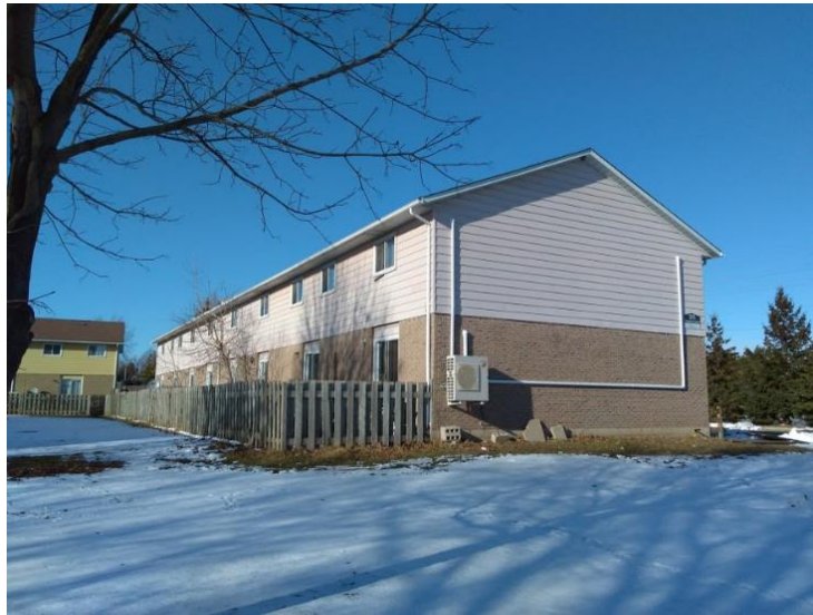
Figure 3-1. Outdoor coil and refrigerant line set for the Mitsubishi heat pump mounted in a 2-bedroom rowhouse end unit.
