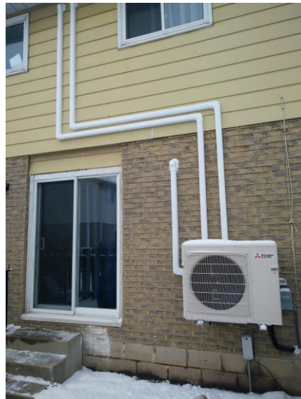
Figure 3-4. Outdoor coil and refrigerant line set for the Mitsubishi heat pump installed in a 3-bedroom rowhouse unit.
