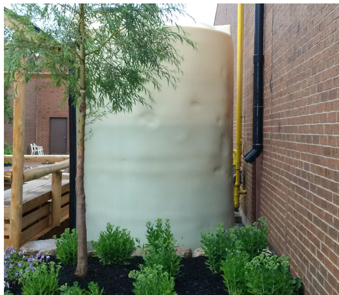
Figure 6. Cistern and disconnected downspout at Calstone
