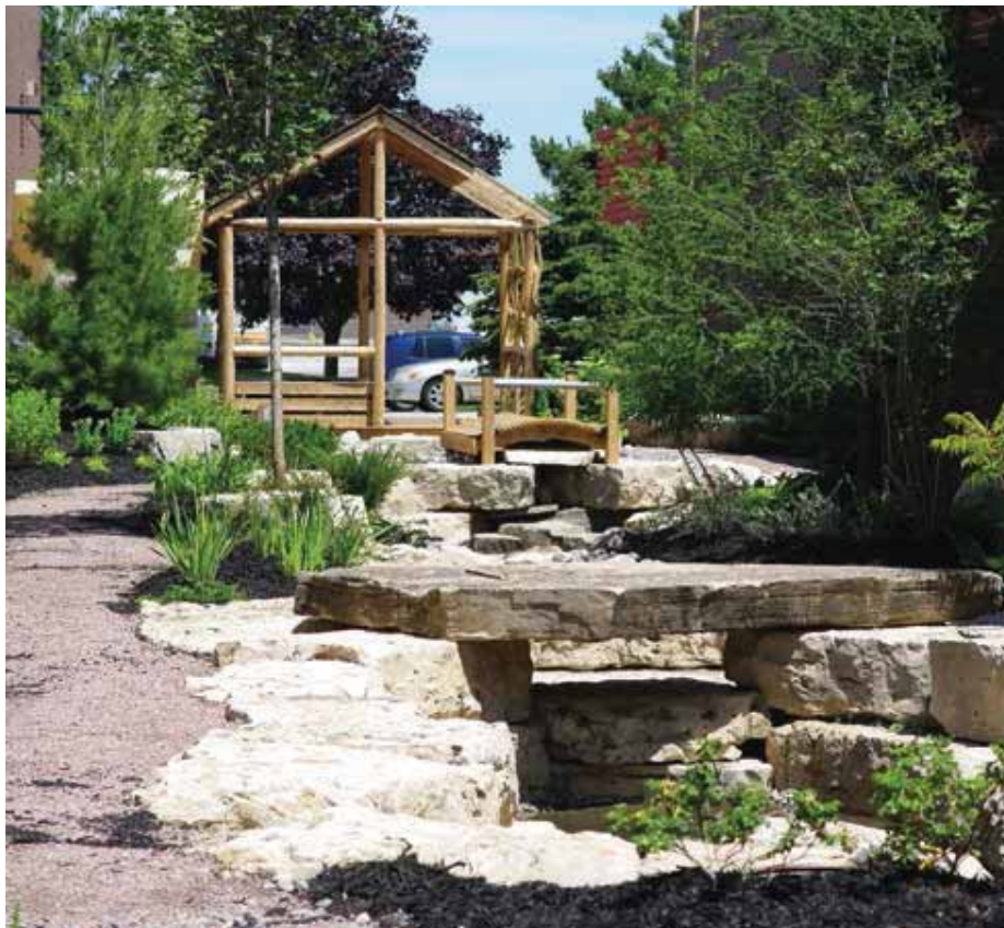
The interconnected stormwater detention and infiltration ponds on Calstone's property. The pond closest to the parking lot acts as spillover from Calstone's rainwater harvesting tank as well as a permanent, attractive water feature. Image by Partners in Project Green
