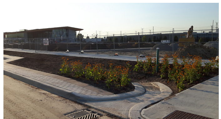
Figure 2. Inlet to bioretention area (Image courtesy of the City of Markham)
