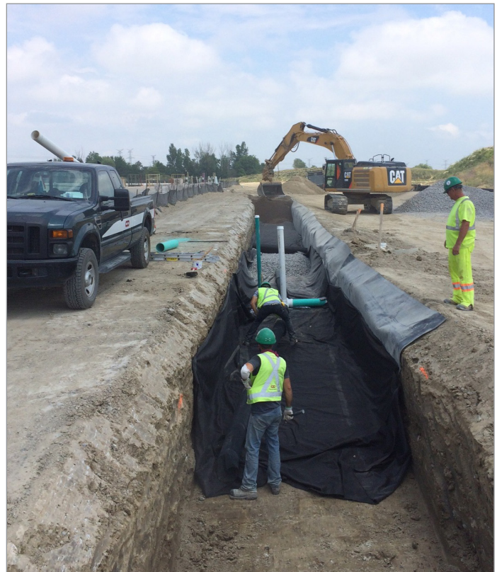
Figure 4. Infiltration gallery construction at the Green Road (image courtesy of City of Markham)
