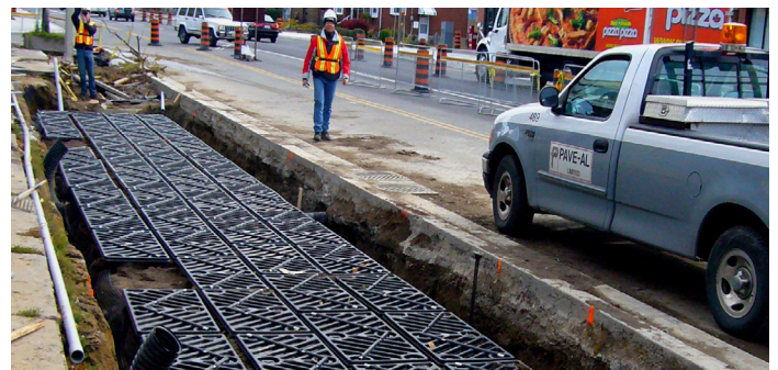
Figure 2. Silva Cell "top" deck prior to organic layer and screenings for pavers. (Image courtesy of City of Toronto)
