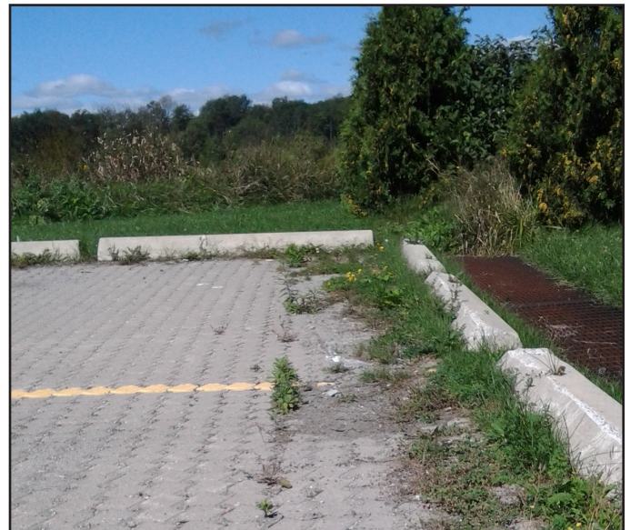
Figure 4. Permeable pavements in needs of maintenance
