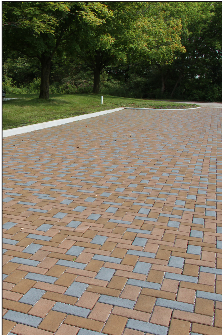
Figure 5. Permeable interlocking recycled rubber composite pavers in a parking lot
