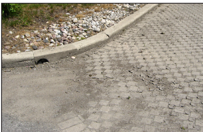
Figure 3. Sediment accumulation on permeable pavement
