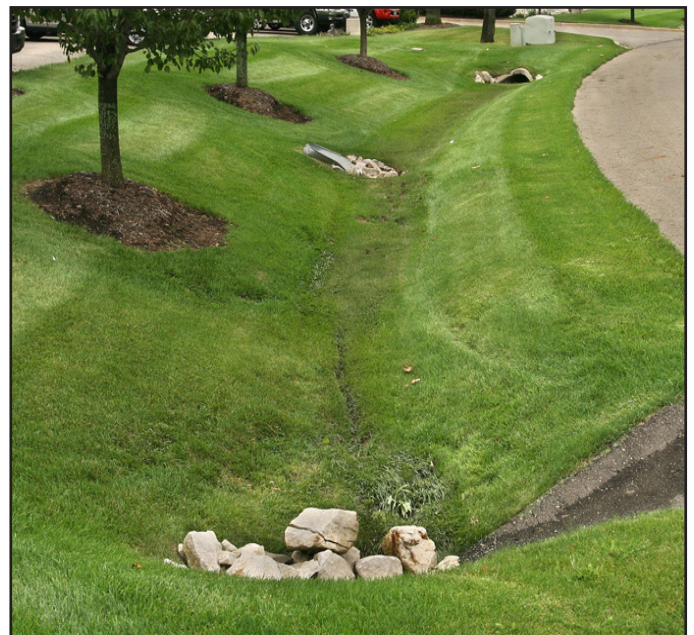
Figure 3. Enhanced swale with stone cover at inlets
