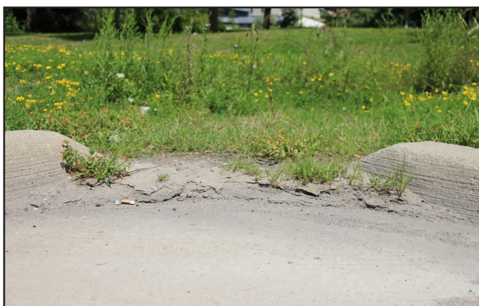
Figure 5. Sediment accumulation at the curb cut inlet to an enhanced swale
