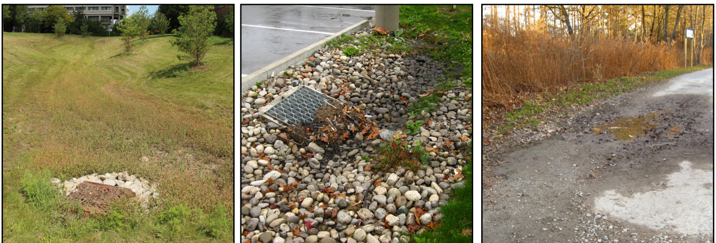
Figure 2. Outlet (left) and inlets (middle and right) in need of maintenance
