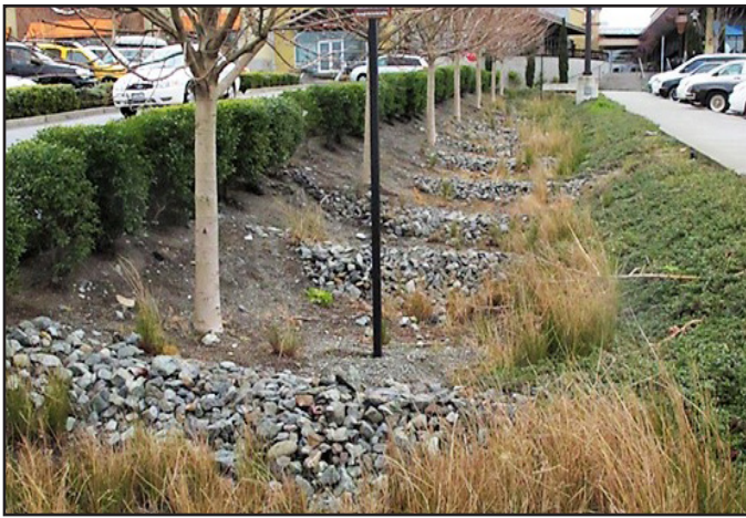
Figure 1. Enhanced swale with check dams (Image courtesy of M. Smith)
