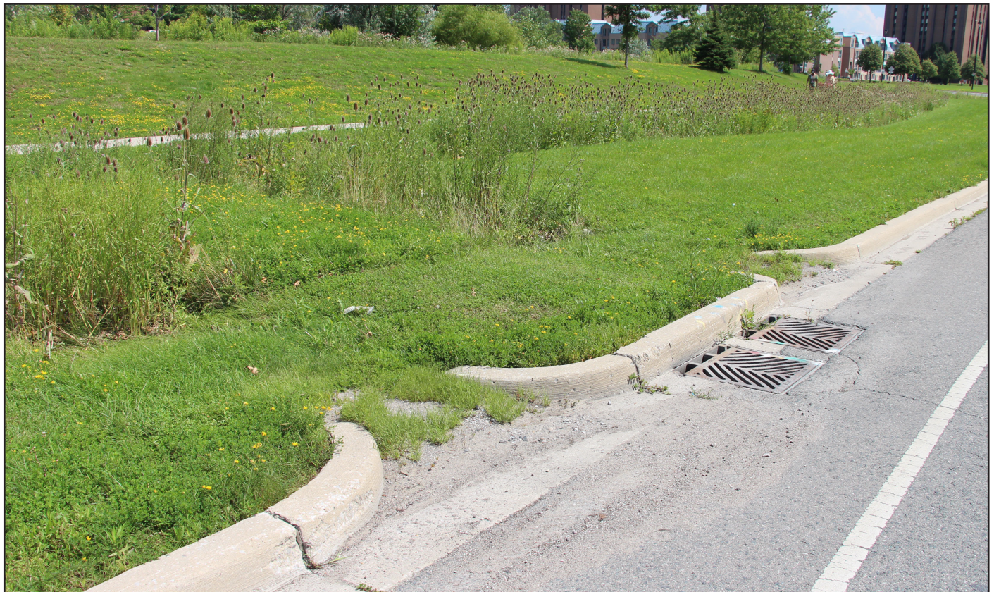
Figure 4. Inlets in need of maintenance due to sediment accumulation
