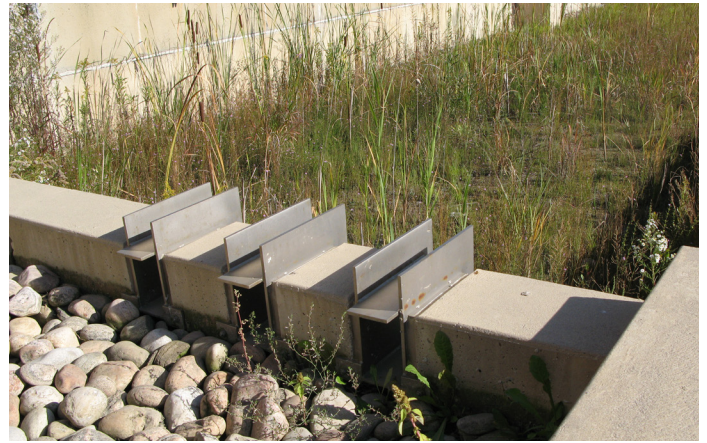
Figure 5. Forebay and inlet to linear wetland feature
