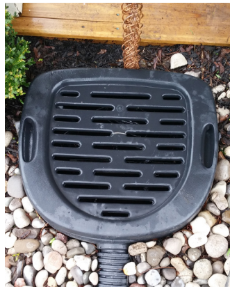
Figure 3. Roof runoff catchbasin
