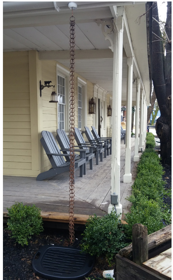
Figure 2. Roof runoff enters the system via rain chains to a small catchbasin
