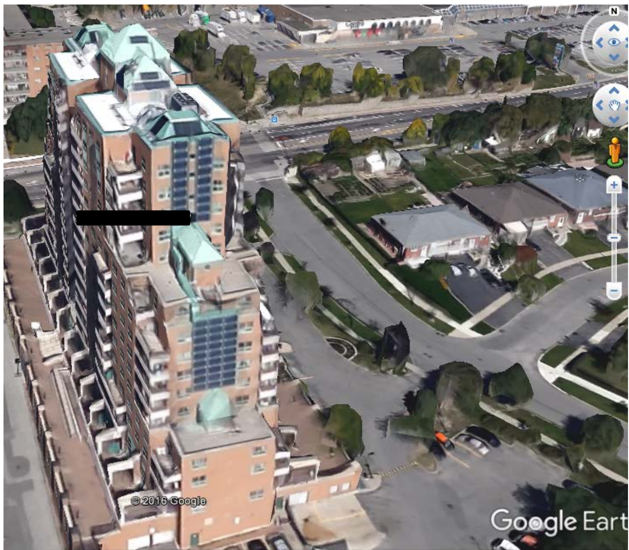
Figure 3-16. With the aid of satellite imagery, the annual energy yield of the PV system at this building was estimated to be 7,800 [kWh].
