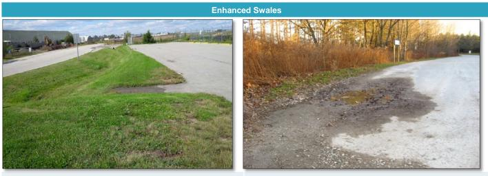
**PASS:** CDA has not changed in size or land cover. Sediment, trash or debris is not accumulating and point sources of contaminants are not visible.
