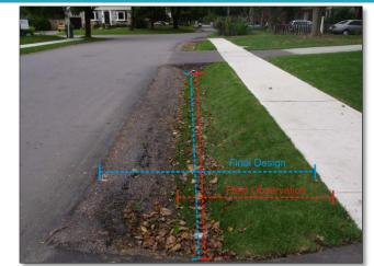
FAIL: The footprint area of the swale is significantly smaller than what was specified in the final design due to half the width having been paved over.
