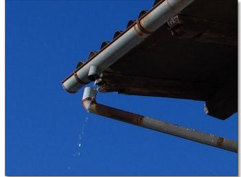
**FAIL:** The roof downspout is disconnected from the eavestrough, preventing runoff from entering the cistern.
