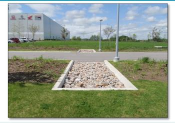
**PASS:** Geotextile-lined stone inlet is free of sediment, trash and debris. Stones to slow down and spread out inflowing water remain in place.
