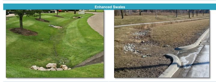
**PASS:** There are no signs of excessive sediment accumulation on the surface of the swale. (Source: DAA)
