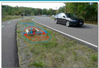
**PASS:** The overflow outlet elevation and maximum surface ponding area closely match what was specified in the final design.
