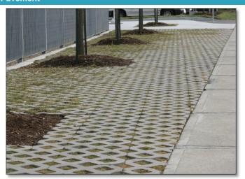
**FAIL:** The turf grass cover on the permeable walkway is not thriving in some areas and needs cutting in others.
