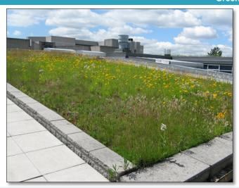
**PASS:** There are no bare areas or signs of erosion of growing media from concentrated flowing water or wind scour on the green roof (i.e. filter bed) surface.
