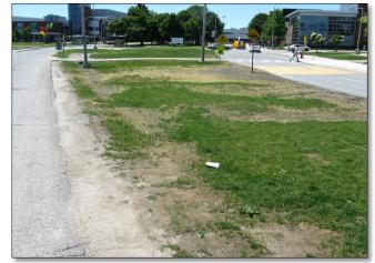
**FAIL:** Presence of large patches of dying vegetation and bare soil indicate that surface ponding occurs regularly and that the vegetated filter strip does not drain well.
