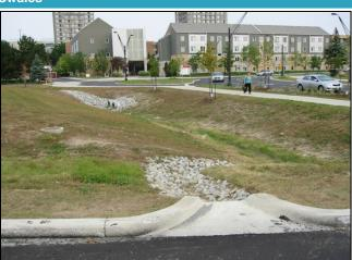
**FAIL:** Major portions of the swale surface contains dead or dying vegetation which reduces its aesthetic value and could be negatively affecting its stormwater treatment function.
