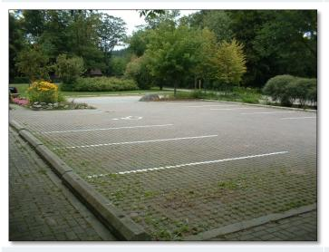
PASS: No damage, displacement or sinking of the permeable surface is visible. Some grass and weeds are growing in the joints between pavers but the affected area is not extensive.
