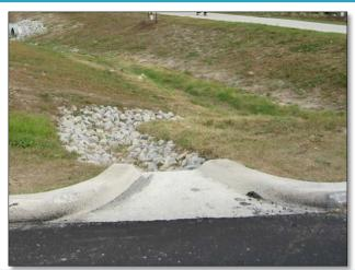
**PASS:** There is no evidence of damage or displacement of the inlet structure and no erosion gullies on the filter bed.
