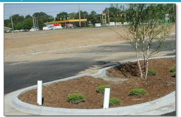
**FAIL:** Size of the CDA has changed from design assumptions. A point source for contaminants is visible (i.e. lack of sediment controls on adjacent construction site). (Source: NCCE)
