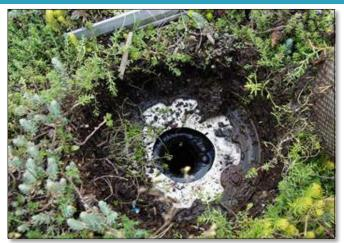
FAIL: Sediment is accumulating at the overflow outlet which could impair its drainage function and cause surface ponding and vegetation die-off. (Source: Jorg Breuning)
