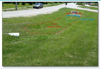
**FAIL:** The elevation of the overflow outlet is higher than what was specified in the design, producing a much larger surface ponding area than intended which could produce standing water for prolonged periods and cause vegetation to die off.
