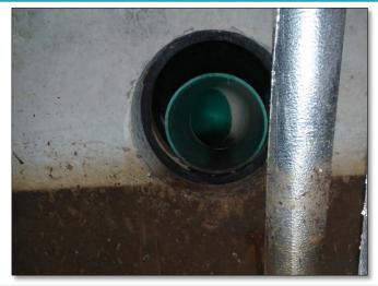
**PASS:** The overflow outlet pipe diameter matches what was specified in the final design and is free of damage and obstruction.
