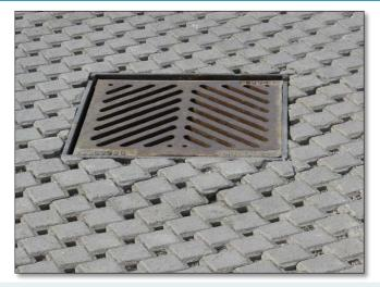
**PASS:** The overflow outlet is free of damage and obstruction and functions as designed to safely convey excess water from the BMP.
