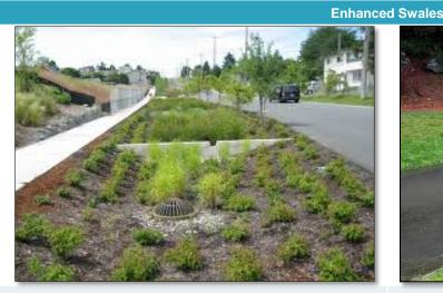
**PASS:** The maximum surface ponding depth behind check dams matches what was specified in the final design. (Source: NEOSWTC)
