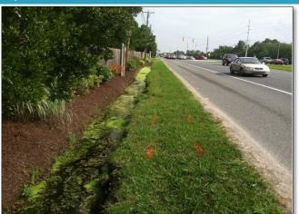
**FAIL:** There is standing water and highly saturated soils on the surface of this dry swale. Presence of algae indicates the swale does not drain between storms. (Source: James Urban).
