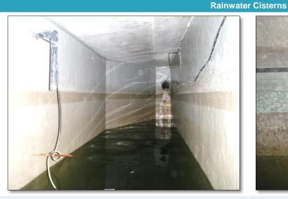
**PASS:** There are no cracks or leaks visible in the cistern structure.
