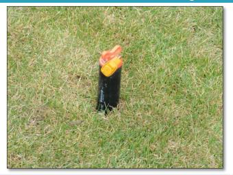
**PASS:** The well is undamaged and accessible and the cap is in place and secured to prevent unauthorized access.
