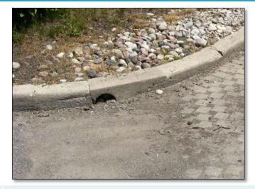
**FAIL:** The overflow outlet is obstructed with sediment which impairs its function to convey excess water from the BMP.
