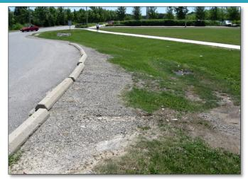
FAIL: Concrete barriers are preventing stormwater from entering the BMP as sheet flow from the pavement. Sediment has accumulated at the inlet edge of the BMP.
