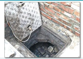
**FAIL:** The access hatch of this cistern was paved over with concrete and ladder rungs are missing which prevents safe entry for inspection and maintenance tasks. (Source: Miles Golding).
