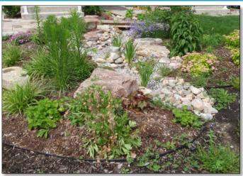
PASS: There is no trash in or around the bioretention area that could possibly block inlets and outlets.
