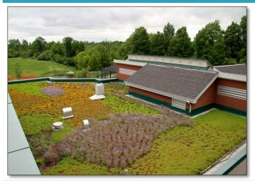
**PASS:** The green roof is well covered by dense, attractive vegetation which helps maintain its stormwater treatment function and aesthetic value. (Source: Earth Rangers)
