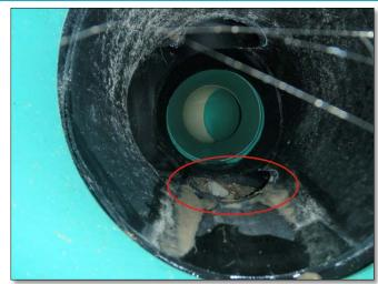
**FAIL:** Sediment has accumulated in the inlet pipe to the infiltration trench and is fully obstructing flow of stormwater into the BMP.
