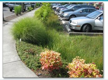
**PASS:** The planted portion of the bioretention cell is completely covered with dense, attractive vegetation which helps to maintain its stormwater treatment function and aesthetic value.
