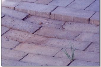
FAIL: The pavement surface has sunk in local areas, creating a trip hazard and the potential for further damage from snow plowing. (Source: Basalite)
