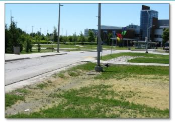
**FAIL:** Scour erosion along the inlet edge is visible. Bare soil areas and bright green biofilm on the filter strip surface indicate that concentrated flow and surface ponding occurs regularly.
