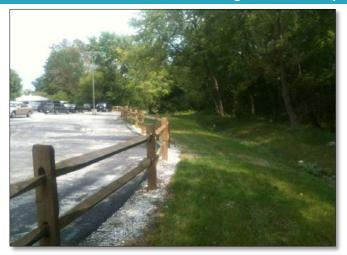
**PASS:** There are no obstructions at the inlet and stormwater can freely flow into the BMP as sheet flow from the pavement and gravel diaphragm. (Source: CSN).
