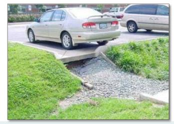
FAIL: Excessive erosion at the inlet is visible and undermining the integrity of the adjacent pavement. (Source: CSN)
