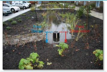
**PASS:** The maximum surface ponding depth of the bioretention cell matches what was specified in the final design.
