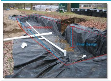
**PASS:** The footprint area and depth of the bioretention cell does not significantly deviate from the final design and should not negatively affect its stormwater management treatment performance.
