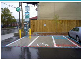
**PASS:** The footprint area of the BMP does not significantly deviate from the final design and should not negatively affect its stormwater management treatment performance.
