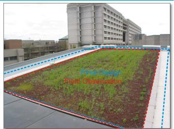
**FAIL:** The footprint area of the green roof is significantly smaller than what was specified in the final design.
