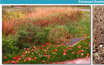
PASS: The overflow outlet of this vegetated swale is free of damage and obstruction and functions as designed to safely convey excess water from the BMP.
