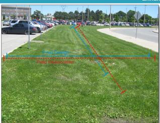
PASS: The footprint area of the BMP does not significantly deviate from the final design and should not negatively affect its stormwater management treatment performance.
