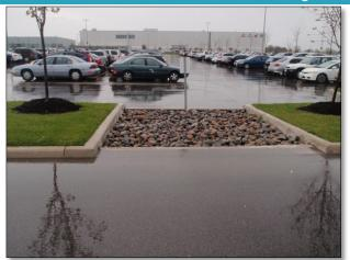
**PASS:** CDA has not changed in size or land cover. Sediment, trash or debris is not accumulating and point sources of contaminants are not visible.
