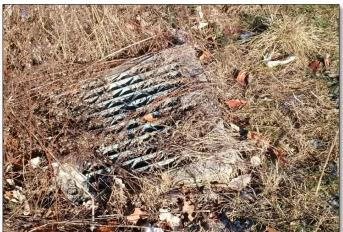
FAIL: Vegetation and debris is partially obstructing the overflow outlet structure which impairs its drainage function .
