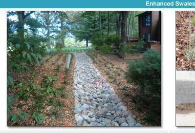
PASS: Mulch depth is within the range specified in the final design (i.e. 5 to 10 cm) and covers all portions of the BMP not covered by stone or vegetation. (Source: Blade Runners)
