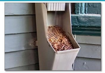
**PASS:** The pretreatment filter of the cistern is free of sediment and debris.
