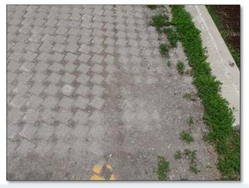
**FAIL:** The joints between pavers are completely filled with fine sediment in local areas and sediment is accumulating on the surface of the pavers.
