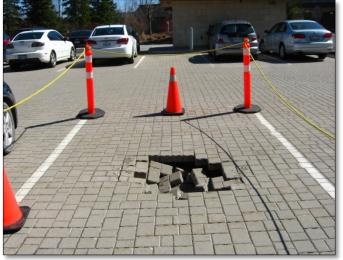
FAIL: A sink hole has formed in one location on the permeable pavement surface, requiring structural repair.
