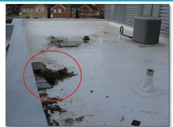
**FAIL:** Accumulated sediment and debris is blocking inflow over greater than one third of the inlet width and preventing stormwater from freely entering the BMP.
