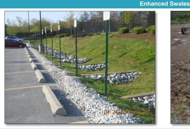
**PASS:** The check dams are visible and continue to help retain sediment and spread the flow of water across the BMP surface. (Source: CSN).
