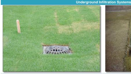
**PASS:** There is no evidence of damage or displacement of the inlet that would prevent runoff from freely entering the BMP.
