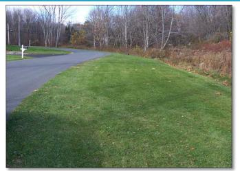
**PASS:** The vegetated filter strip is evenly covered with dense turf grass which helps to maintain its stormwater treatment function and aesthetic value. (Source: Trinkaus Engineering)
