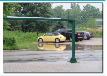
**PASS:** CDA has not changed in size or land cover. Sediment, trash or debris is not accumulating and point sources of contaminants are not visible.
