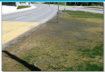
**FAIL:** Size of the CDA or land cover within it has changed from design assumptions. Accumulation of sediment on the CDA is visible.
