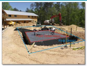
**FAIL:** The size of the cistern being installed is much smaller than what was specified in the final design.
