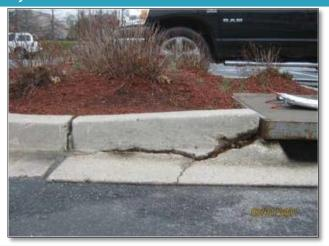
FAIL: The inlet structure has been damaged or displaced and requires repair. (Source: CSN)
