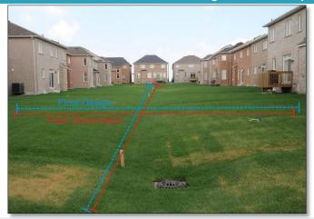
**PASS:** The footprint area where soil amendments have been implemented does not significantly deviate from the final design and should not negatively affect its stormwater management treatment performance.
