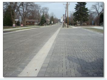
**PASS:** No portion of the pavement is covered in sediment and fine gravel fill material within the joints between pavers is still visible.
