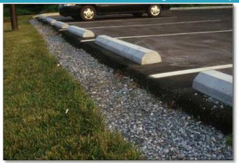
**PASS:** There is no evidence of damage to the gravel diaphragm inlet that would prevent runoff from entering the BMP nor excessive erosion of the filter bed. (Source: Aquafor Beech)
