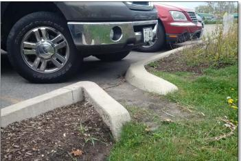
**FAIL:** Accumulated sediment and vegetation is preventing stormwater from entering the BMP. Sediment on the pavement surface in front of the inlet indicates ponding is occurring.
