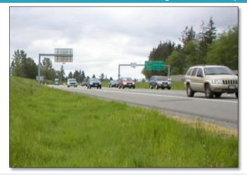
**PASS:** There is no standing water on the vegetated filter strip and no bare soil areas that would indicate surface ponding occurs regularly. (Source: Washington State DOT)
