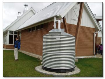
**PASS:** Inlet pipe and couplings are securely connected to the CDA and cistern. (Source: Lake County SMC)
