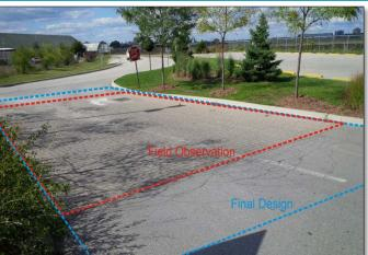
**FAIL:** The footprint area of the BMP is significantly smaller than what was specified in the final design.
