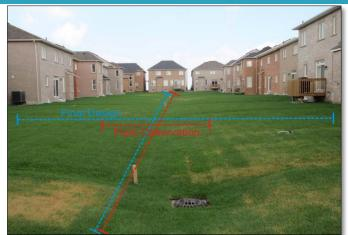
**FAIL:** The footprint area where soil amendments have been implemented is significantly smaller than what was specified in the final design.
