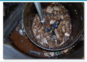
**FAIL:** Accumulated sediment, trash and debris in the hydrodynamic (i.e., oil and grit) separator is occupying greater than 50% of its storage capacity. (Source: SWC Canada)
