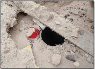
**FAIL:** The well has been left uncapped and unprotected from erosion and sediment during construction.
