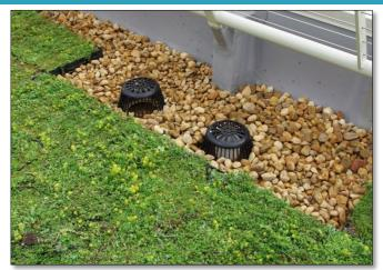
**PASS:** The overflow outlets of this green roof are free of damage and obstruction and function as designed to safely convey excess water from the BMP. (Source: Vegetal I.D.)
