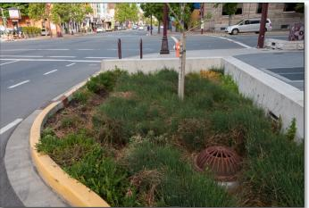
PASS: The overflow outlet is free of damage and obstruction and functions as designed. (Source: Dylan Passmore)
