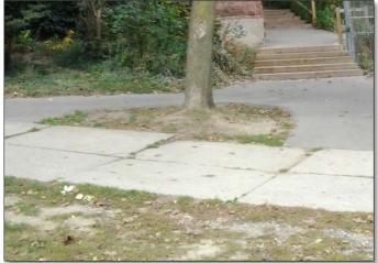
**FAIL:** Major portions of the filter strip contain bare soil or dead vegetation which reduces its aesthetic value and could be negatively affecting its stormwater treatment function.
