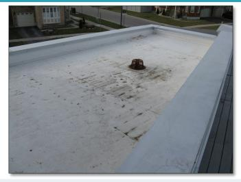
**PASS:** There are no obstructions at the inlet and stormwater can freely flow into the BMP
