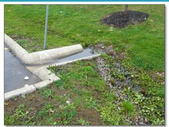
**FAIL:** Erosion gullies and bare soil areas are visible on the swale surface at the inlet.
