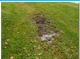
**FAIL:** Clear evidence of bed sinking is visible, creating a preferential ponding area where vegetation has died off.
