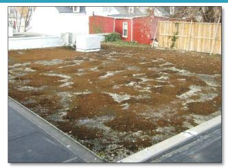
**FAIL:** Standing water is present on the green roof surface and in the sub-drain system and bare soil areas are visible. (Source: J.V. Heidler)
