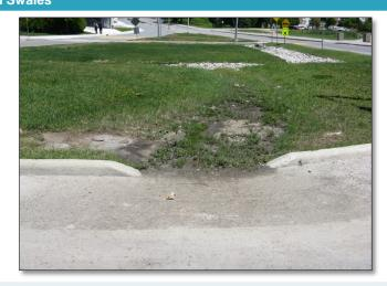
**FAIL:** Accumulated sediment and vegetation is preventing stormwater from entering the BMP. Sediment on the pavement surface in front of the inlet indicates ponding is occurring.
