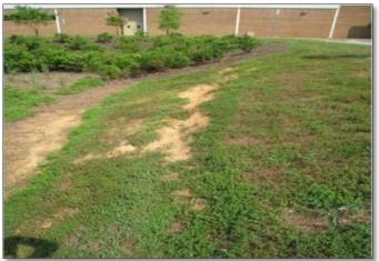
**PASS:** No erosion gullies, bare soil areas or ruts are visible on the side slopes. (Source: City of Maplewood)
