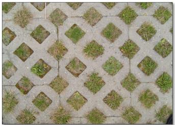
**FAIL:** The vegetation cover on the permeable pavement is a mixture of turf grass and invasive species (i.e. weeds). (Source: Immanuel Giel)
