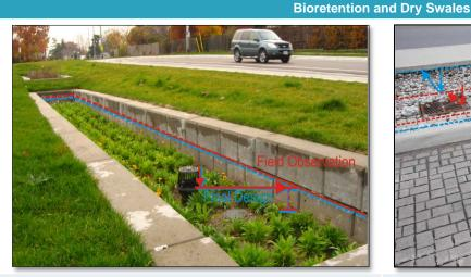
**PASS:** The overflow outlet elevation and maximum surface ponding area match what was specified in the final design.
