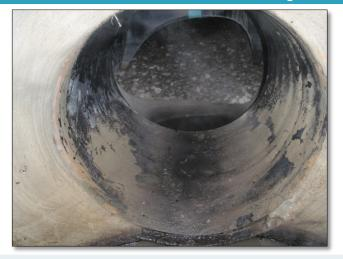
**PASS:** The sub-drain outlet pipe from the infiltration chamber system is not obstructed by sediment, debris or roots and shows no signs of damage.
