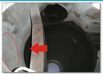
**PASS:** The overflow outlet weir wall and storm sewer pipe in the control manhole of this infiltration chamber system is free of damage and obstruction and functions as designed to safely convey excess water from the BMP.
