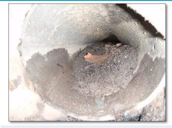
**FAIL:** A perforated pipe in an exfiltration storm sewer system is clogged by sediment and debris which inhibits its drainage function.
