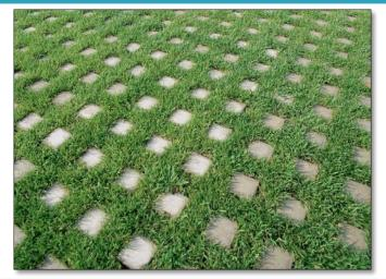
**PASS:** The vegetation cover on the permeable pavement is turf grass as specified in the final design and contains very few weeds. (Source: WEF)
