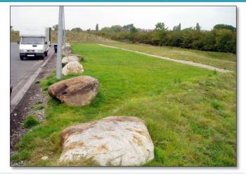
**PASS:** There are no erosion rills, gullies or bare soil areas on the filter strip surface. (Source: CIRIA)
