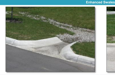
**PASS:** There are no obstructions at the inlet and stormwater can freely flow into the BMP.
