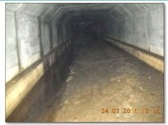
**FAIL:** A substantial amount of sediment has accumulated on the coarse gravel filter bed of the infiltration chamber system which could be impairing the drainage function of the BMP. (Source: Stormwater Maintenance)
