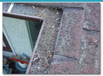
**FAIL:** Sediment and debris is accumulating on the CDA due to deteriorating roof shingles. Eavestroughs need cleaning.
