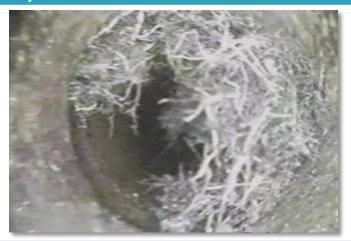
**FAIL:** Roots have penetrated the sub-drain pipe and are substantially reducing its conveyance capacity. (Source: Pipelining Denver)
