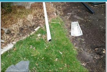
**FAIL:** Splash pad has been displaced and could lead to excessive erosion of the filter bed.
