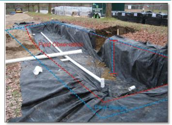
**FAIL:** The footprint area of the bioretention cell deviates significantly from the final design.
