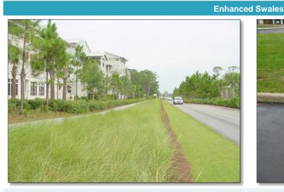
PASS: The grass filter strip pretreatment is free of sediment, trash and debris. (Source: Abbey and Associates).
