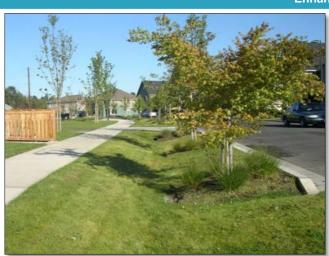
**PASS:** The filter bed has retained its original grading without any sharp depressions that would indicate surface bed sinking. (Source: SVR Design).
