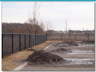
FAIL: Point sources of contamination are present (i.e. accumulated sediment and debris from melted snow piles).
