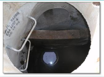
**PASS:** The control manhole of this infiltration chamber system is accessible with ladder rungs in place and no signs of leaking around the weir wall and pipe connections.
