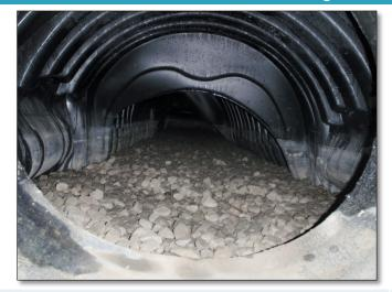
**PASS:** The coarse gravel filter bed of this infiltration chamber system has very little sediment accumulated on the surface indicating pretreatment devices are working well and that sediment removal from the gravel filter bed is not needed.
