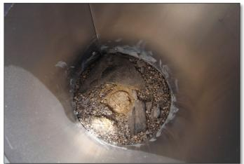
**PASS:** The well is undamaged and accessible and the cap is in place and secured to prevent unauthorized access.
