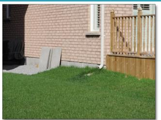
**PASS:** The lawn where soil amendments have been implemented is well graded with no signs of localized bed sinking , animal burrows or ruts.
