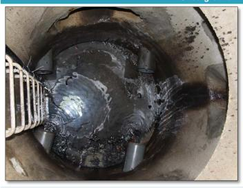
**PASS:** There is some sediment accumulated in the manhole but it is not impairing the flow of stormwater into or out of the BMP. (Source: SWC Canada)
