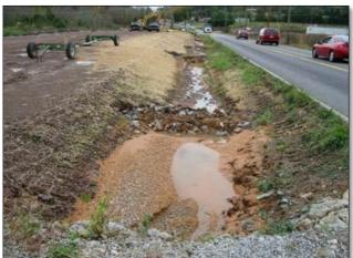
**FAIL:** Sediment has accumulated on the upstream side of the check dam and is affecting its function. (Source: Tennessee EPSC).
