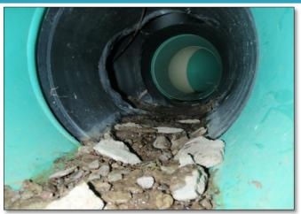
**FAIL:** Sediment and debris has accumulated in the overflow outlet pipe which impairs its function to convey excess water from the BMP.
