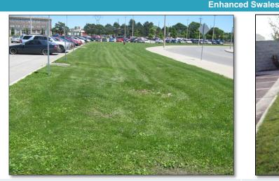
**PASS:** There is no standing water on the surface of the swale and no bare soil areas around the outlet that would indicate surface ponding occurs regularly.
