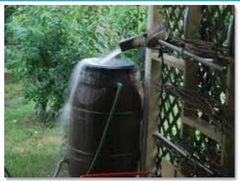
FAIL: The overflow outlet pipe on this rain barrel is undersized and obstructed which impairs its function to safely convey excess water from the BMP. (Source: Melinda Webb)
