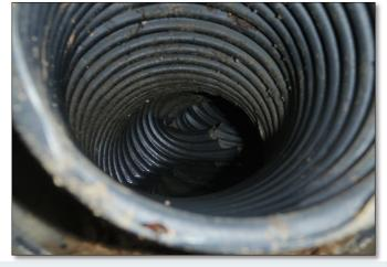
**PASS:** The solid section of the sub-drain pipe is not obstructed by sediment, debris or roots and shows no signs of damage.
