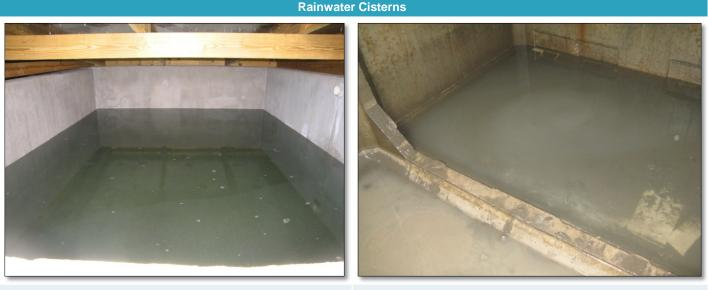
**PASS:** Very little sediment and no coarse debris has accumulated on the bottom of the cistern and the sediment is not at the level of the distribution system intake structure.
