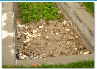
**FAIL:** Sediment accumulation is visible on the filter bed surface and stone covering it and is greater than 5 cm deep.
