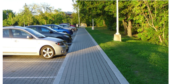
Figure 4. Permeable pavement parking spaces and pedestrian walkways
