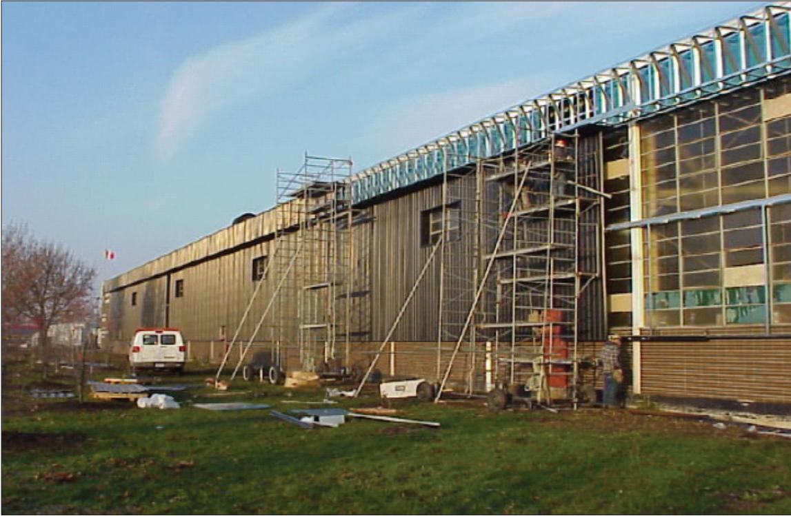
Figure 1. Installation of solar wall.
