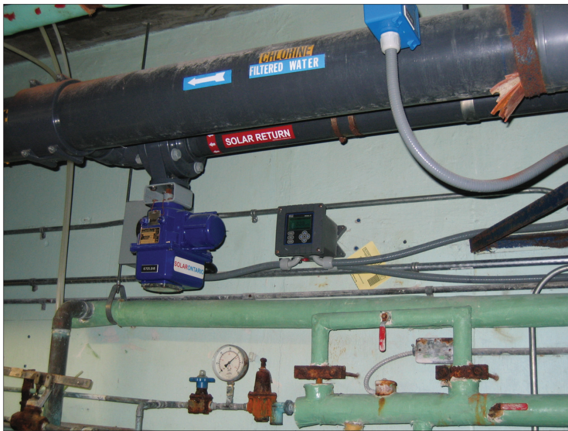
Figure 5. Two-way motorized valve installed on collector return piping.
