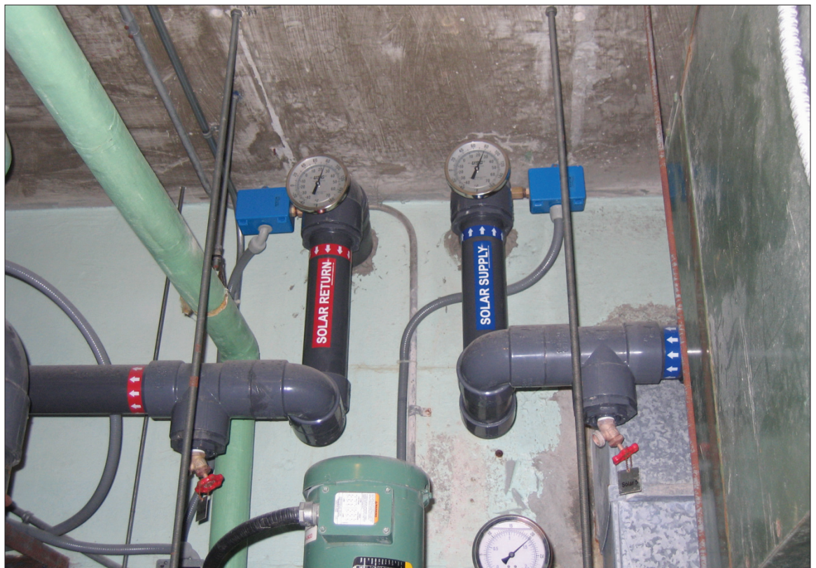
Figure 4. Solar collectors supply and return piping with temperature sensors.
