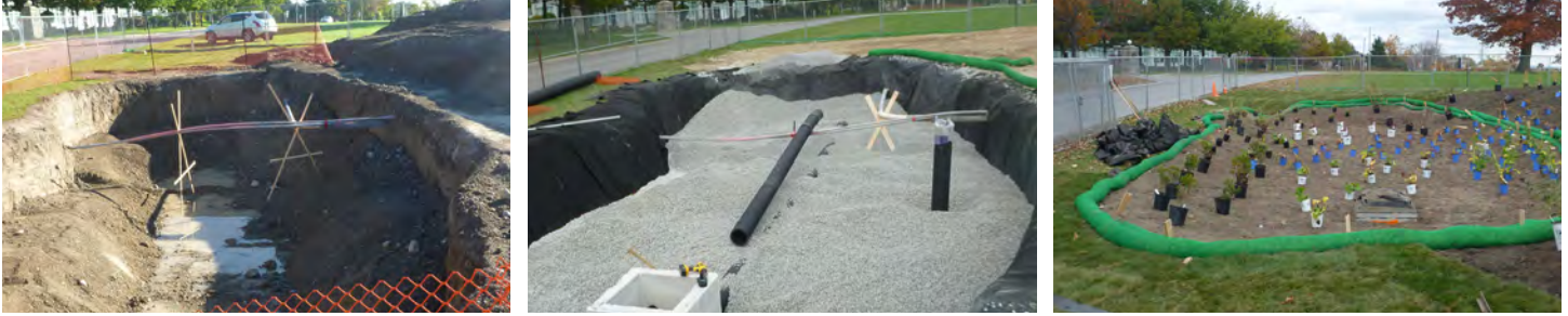
Figure 3. Construction progress at Site 1 (Pictures courtesy of Town of Ajax & Aquafor Beech Ltd.)
