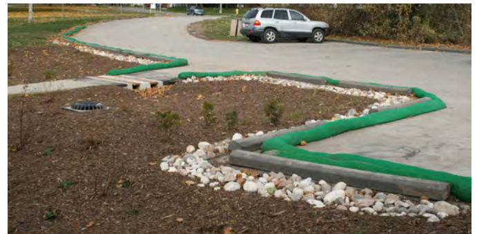
Figure 6. Erosion and sediment control socks protecting Site 2
