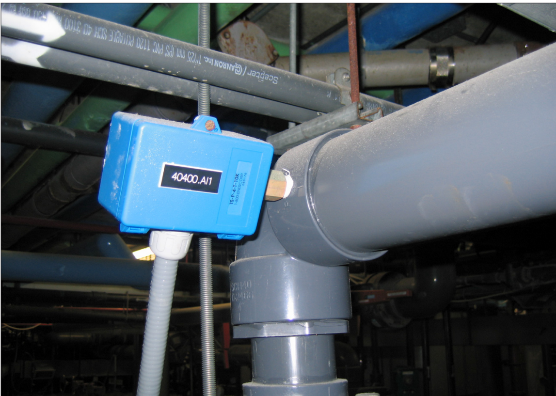
Figure 9. BAS solar heating system temperature sensor
