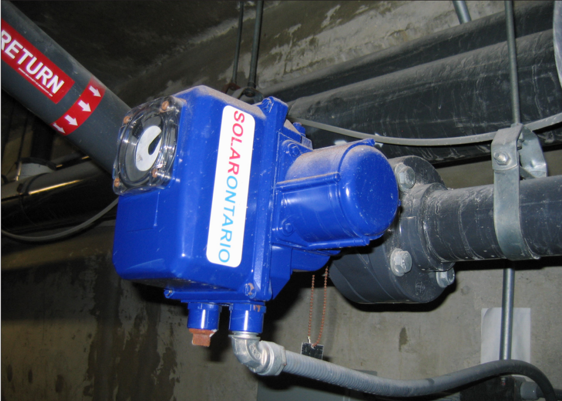
Figure 9. BAS solar heating system temperature sensor
