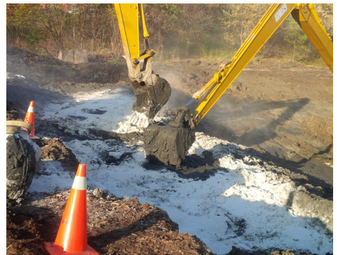
Figure 5. Polymer application using long reach excavators for spreading.
