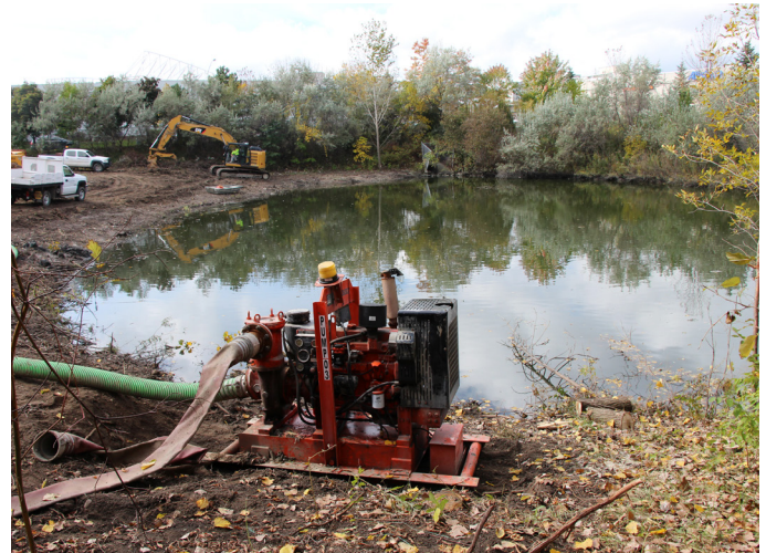
Figure 3. Pumping of Lansing pond.
