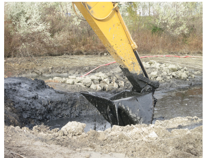
Figure 4. Sediment consistency after dewatering and prior to polymer application.
