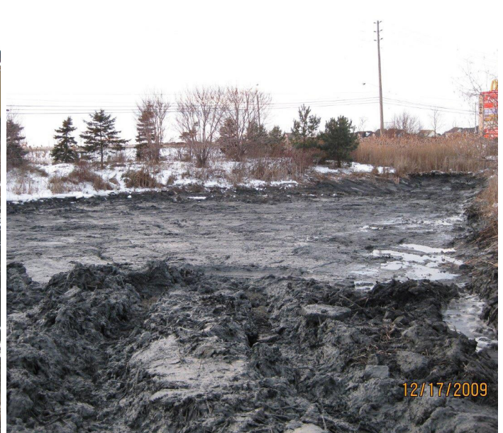
Figure 2. (Left) Excavator removing wet sediment at Pond 51; (Right) Close-up view of the wet sediment at the pond bottom. Sub-zero temperatures have contributed to some freezing of the water-based muck.
