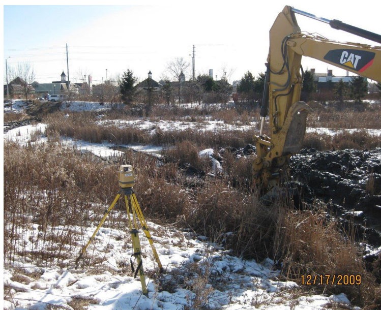
Figure 2. (Left) Excavator removing wet sediment at Pond 51; (Right) Close-up view of the wet sediment at the pond bottom. Sub-zero temperatures have contributed to some freezing of the water-based muck.
