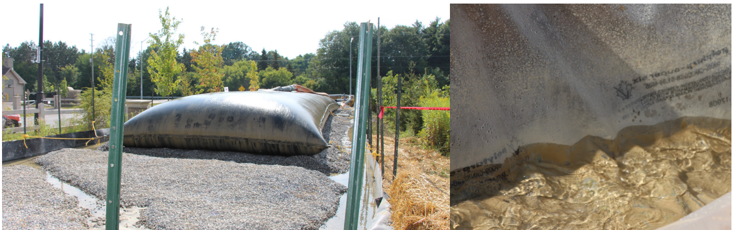
Figure 6. Filled sediment dewatering bag (left) and clarity of effluent water after it drains from the sediment dewatering area (right).
