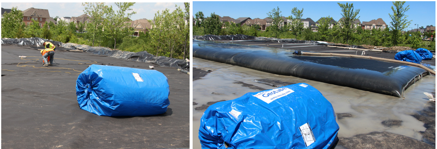
Figure 2. Preparation of laydown area for sediment dewatering Geotubes® (left). The same area with the Geotubes® in place and filtering water (right).
