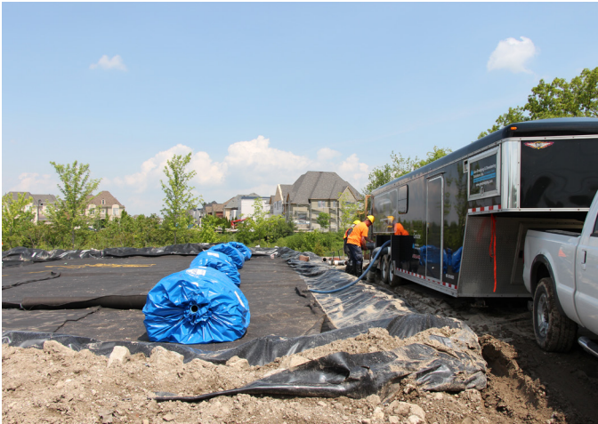
Figure 5. Sediment dewatering bag laydown area.
