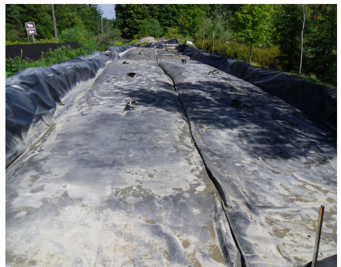
Figure 9. Sediment dewatering bags at the end of dredging.
