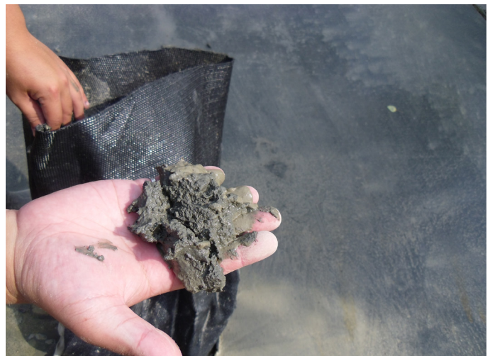
Figure 8. Level of sediment consolidation from within the dewatering bags.
