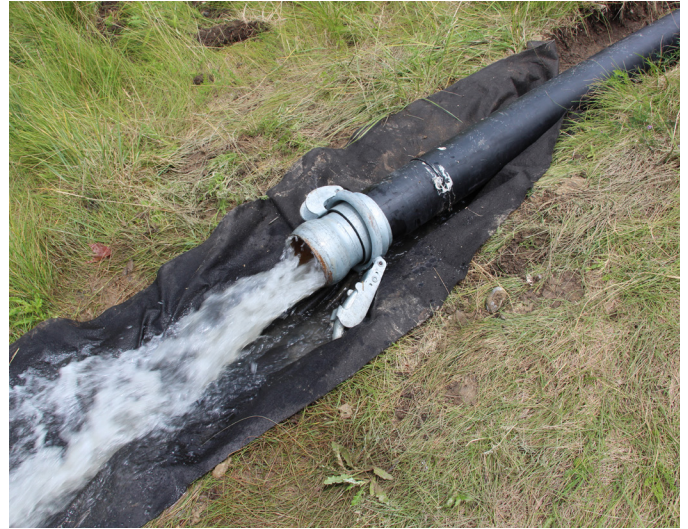
Figure 7. Clear water exiting the sediment dewatering bags.
