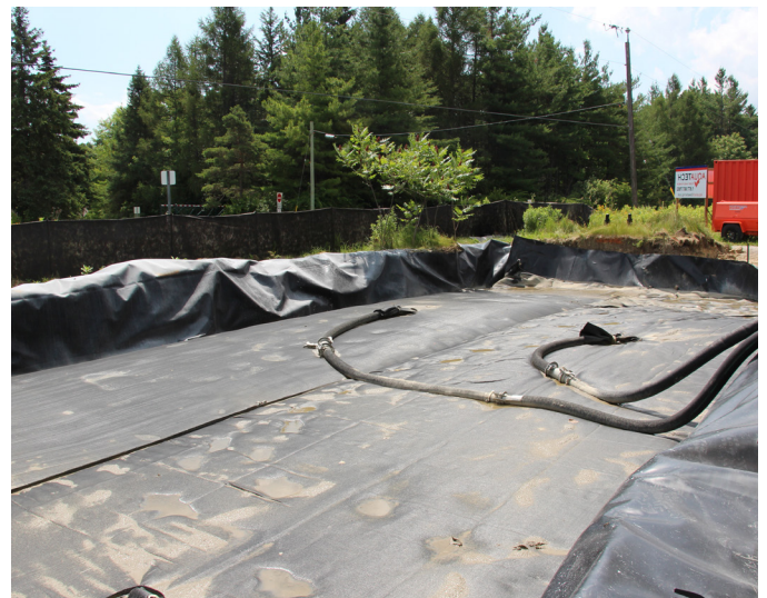
Figure 6. Sediment dewatering bags.
