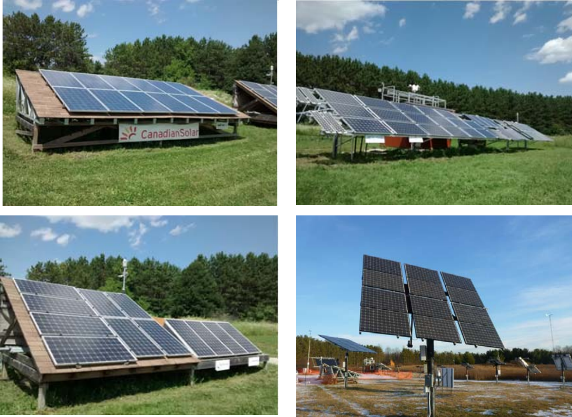
Figure 3.1.2: Travelling clockwise from the top left, example PV arrays connected to Inverters A to D are shown, respectively. In the case of Inverters C and D, there are actually multiple inverters and therefore, those presented here are not exhaustive of all inverters on the property.
