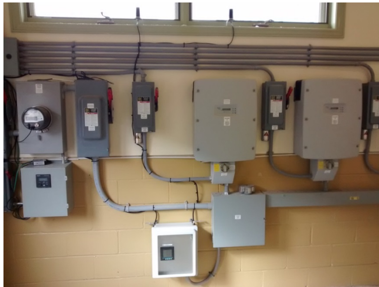
Figure 3.3.3: The monitoring instrumentation is installed to the bottom left of the combiner panel. Current is measured using a Rogowski coil CTs wrapped twice around the wire.
