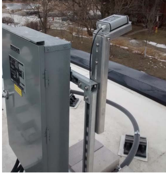
Figure 3.2.3: A plane-of-array irradiance sensor is installed on the roof-top adjacent to the AC combiner panel.
