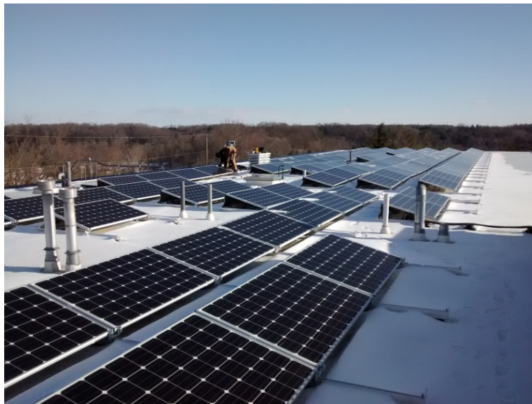
Figure 3.2.1: The Restoration Services Centre facility has a 38.9 kW rooftop PV array.
