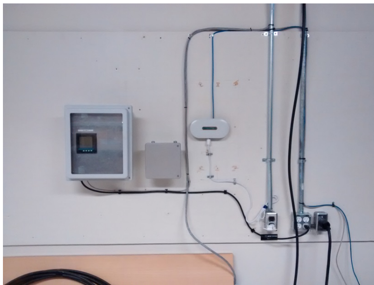
Figure 3.2.4: Sensor wires from the rooftop combiner panel penetrate through the roof to terminate at an instrumentation box mounted indoors.
