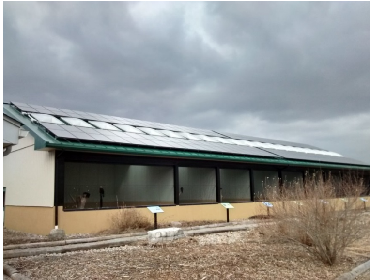
Figure 3.3.1: The Aviary building of the Earth Rangers Centre for Sustainable Technology has a 30 kW rooftop PV installation.
