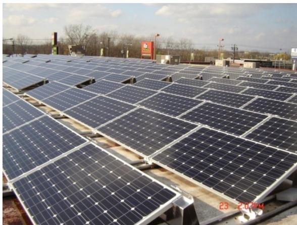
**Figure 2.1.** Site 1 is a 100 kW AC rooftop PV installation in St. Catharines, ON (Photo credit: SolarShare).
