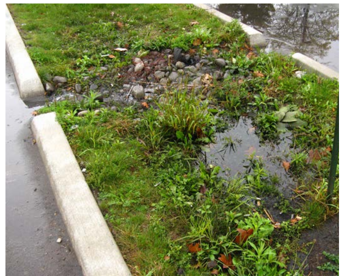
Figure 4. Bioretention inlets in parking lot traffic islands
