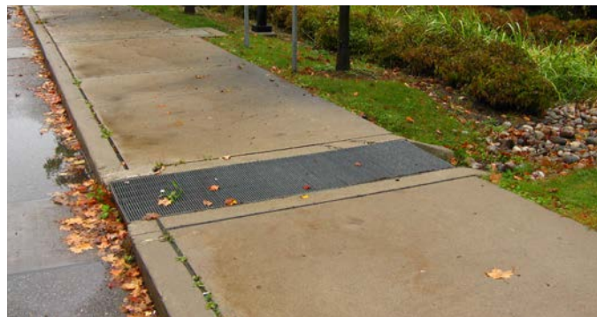
Figure 5. Leaf litter potentially clogging bioretention inlet
