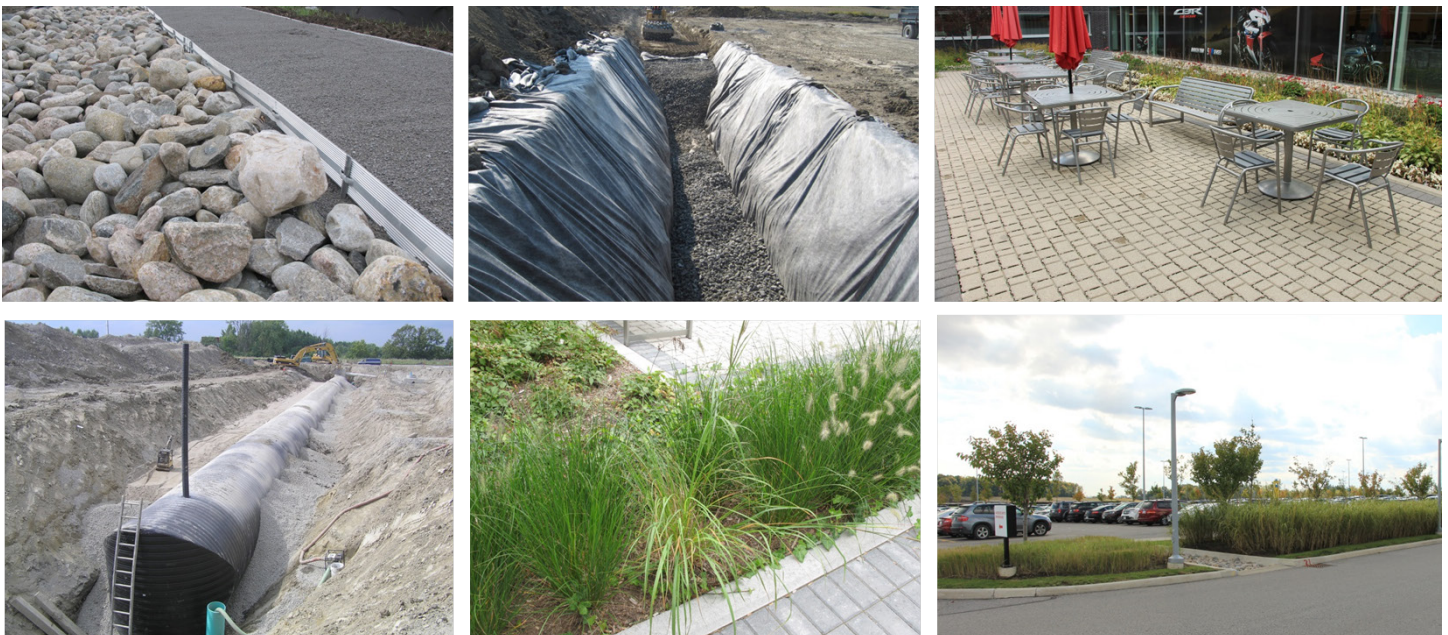
Figure 1. From left to right: Drainage swale and fitness path, biofilter stone trench, permeable surfaces in outdoor eating areas, rainwater cistern, native plantings, vegetated biofilter
