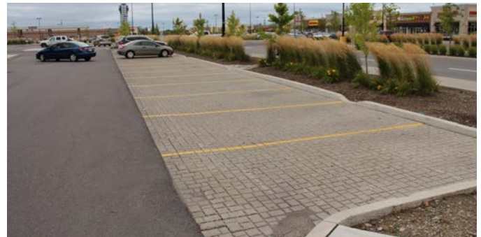
Figure 4. Permeable pavement strip with stormwater biofilter inlets
