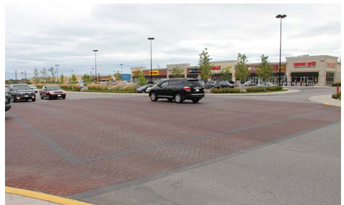
Figure 2. Permeable pavement section in parking lot away from store fronts
